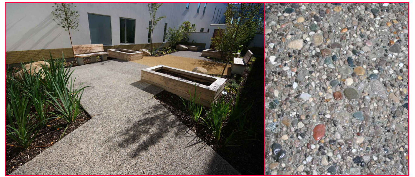
Exposed aggregate concrete paving
