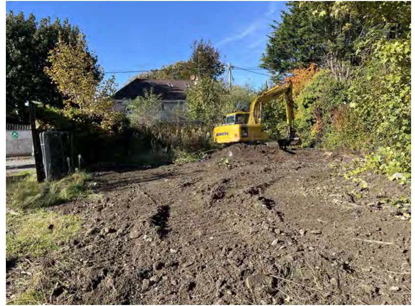
Plate 21: Backfilling of trenches 5 & 8, facing west.
