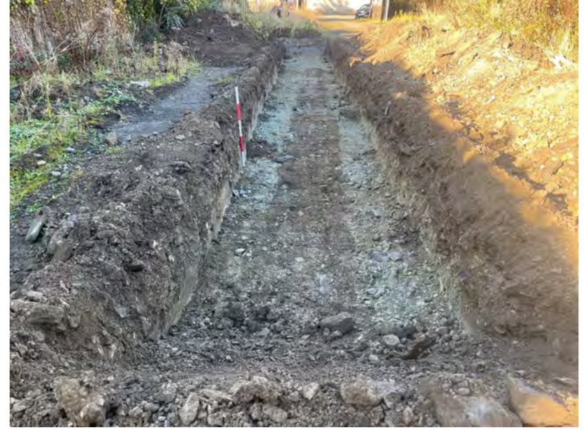
Plate 17: Trench 7 with linear ditch for modern plastic pipe, facing west.
