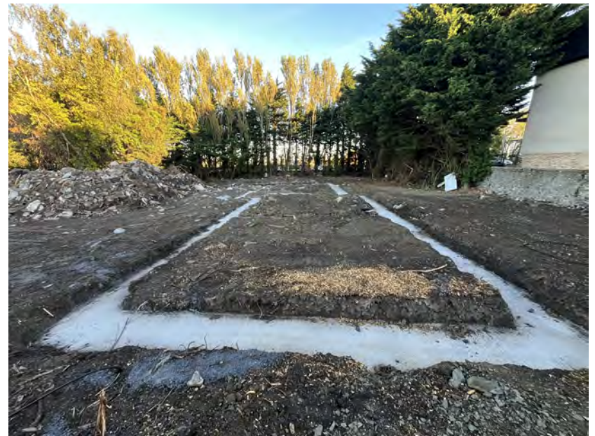
Plate 11: Area of Trench 4 with new concrete foundations, facing north.
