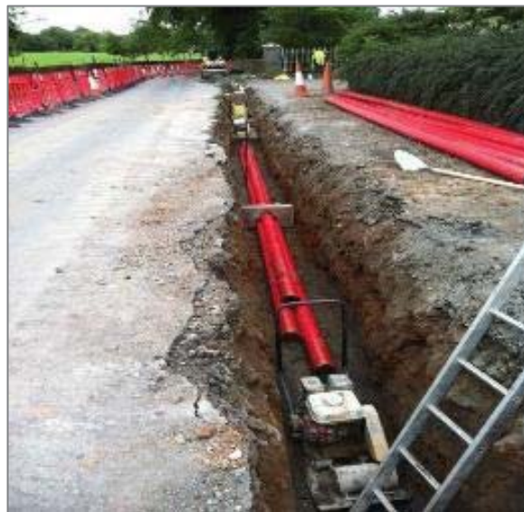
Fig 3.5.1. Example of 110kV Underground Duct installation
