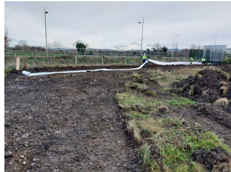
Plate 4: Topsoil stripping at the edge of construction site, facing east
