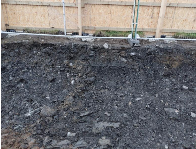
Plate 5: Topsoil stripping at the edge of construction site, facing north
