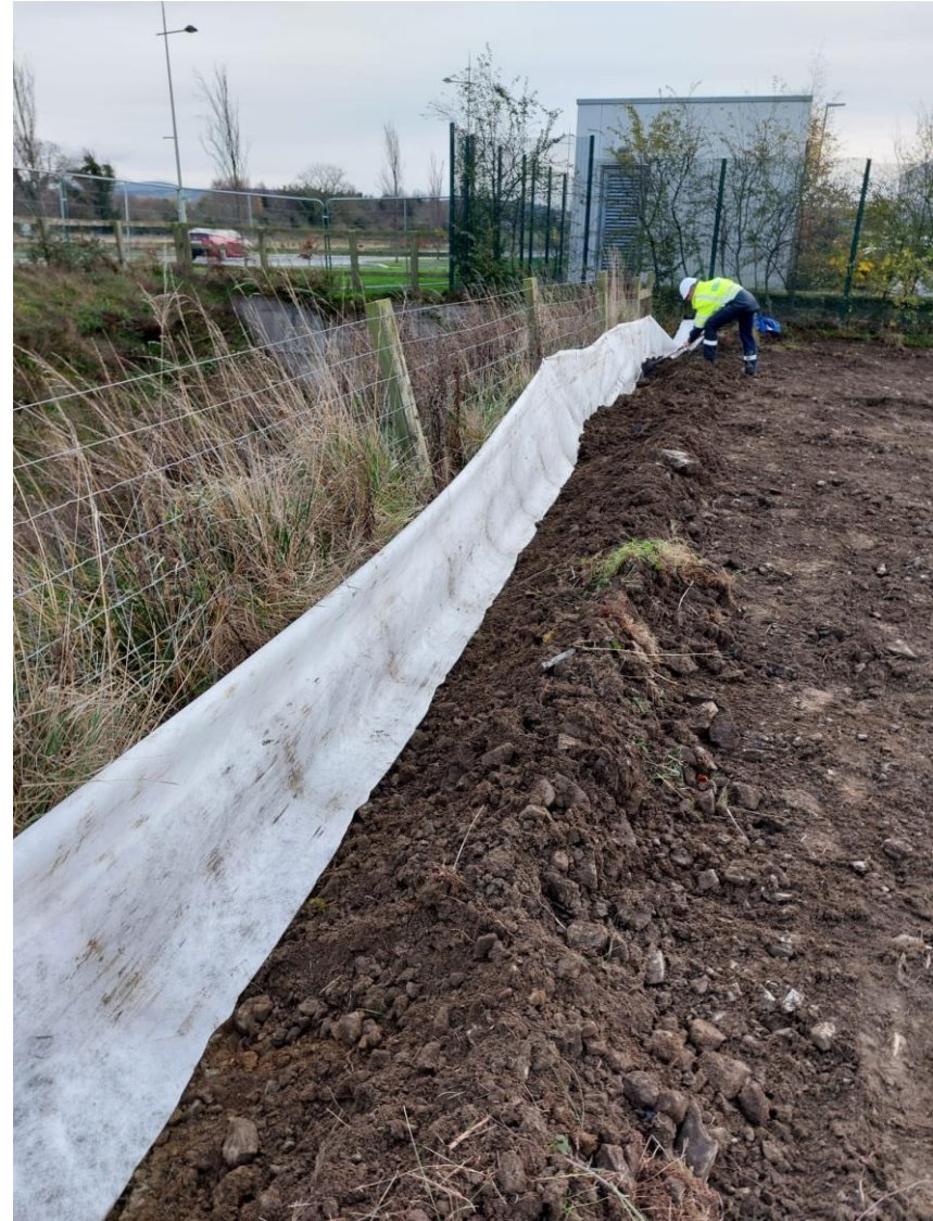
Plate 6: Topsoil stripping at the edge of construction site, facing south
