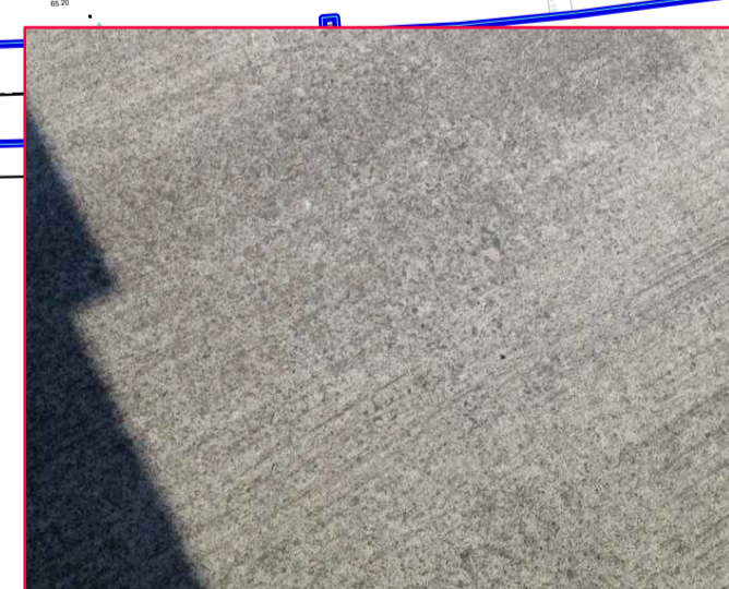
Brushed concrete paving
