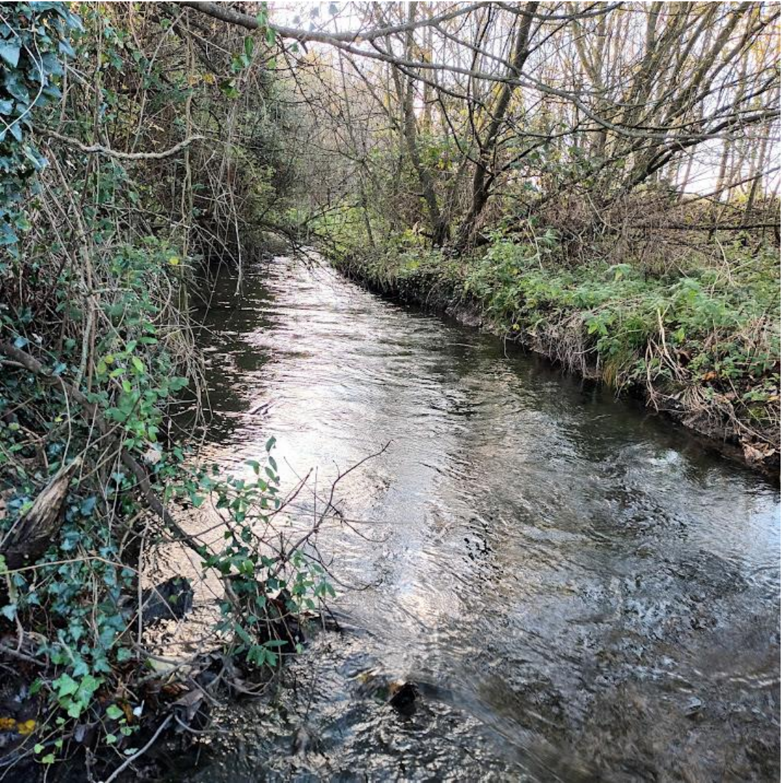
Watercourse and bridge to the south
