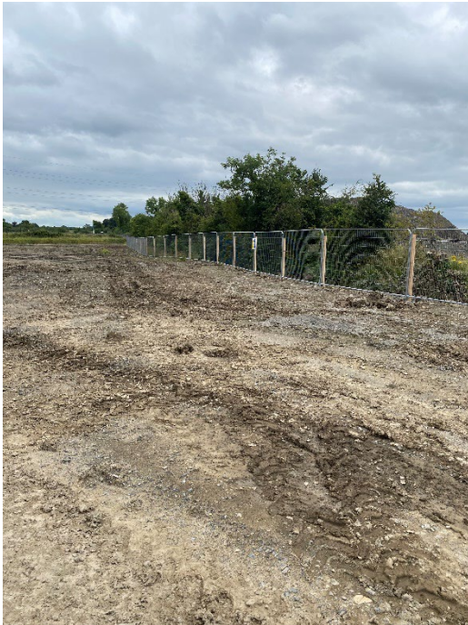
Hedgerow Protection and signage now in place 3
