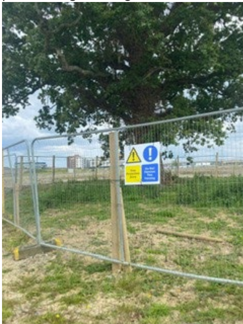
Protective fencing now in place around oak tree. Note signage also in place.
