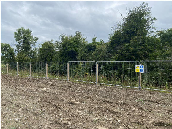
Line of protective fencing reinforced with timber stakes and concrete base
