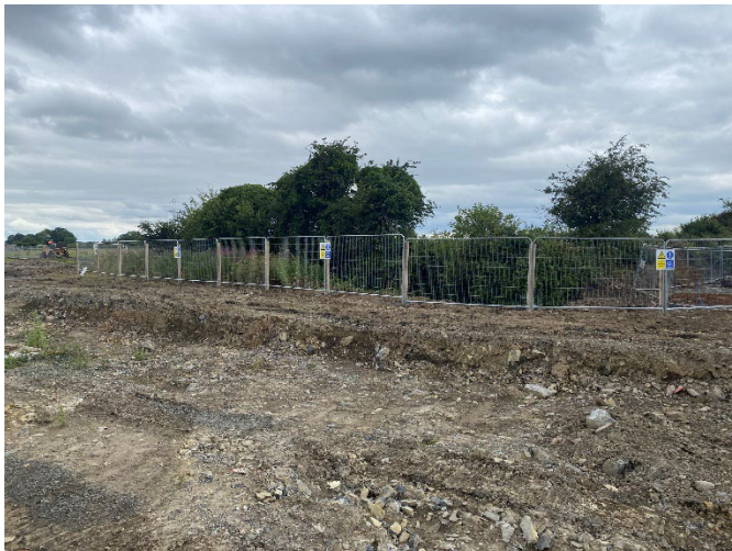
Hedgerow protection and signage now in place 2
