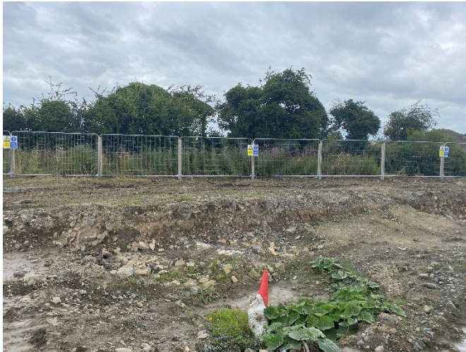
Hedgerow protection and signage now in place 1
