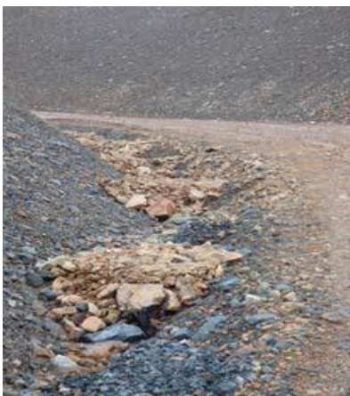
Photo 1 Typical Gravel trap arrangement
