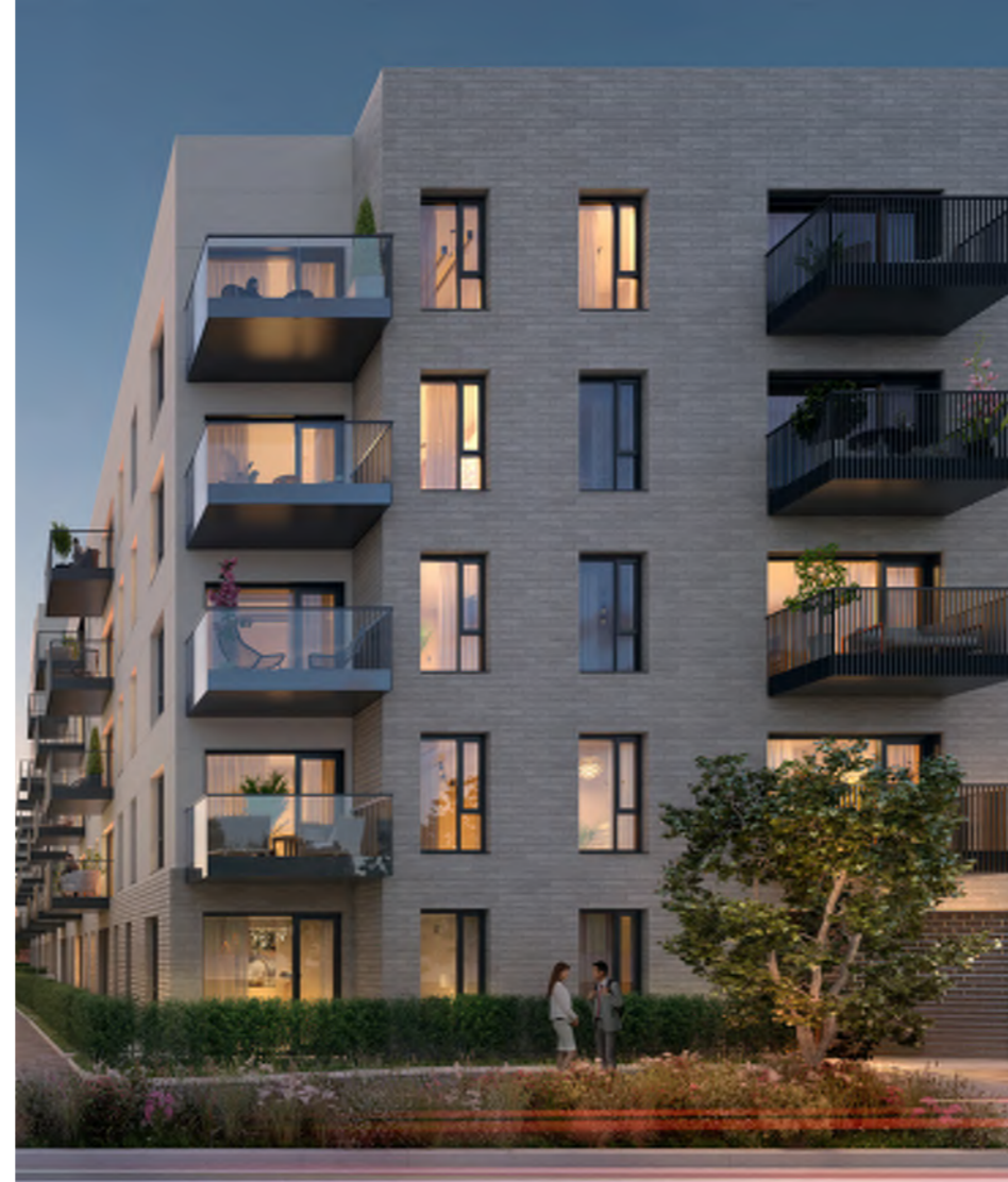
BLOCK C - FROM STATION ROAD
