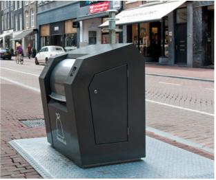
Cardboard compactor in Amsterdam with an Amsterdam column, Kinshofer lifting mechanism and briefcase inlet of 400mm x 150mm.
