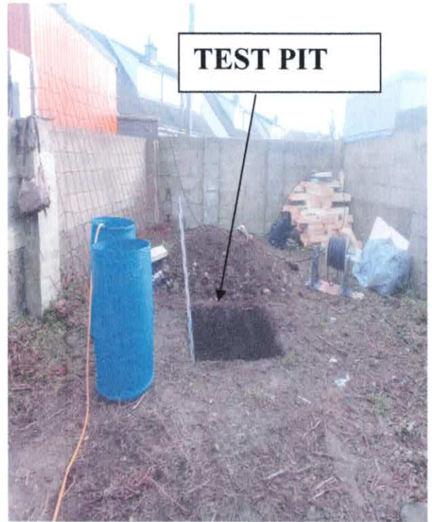
TEST HOLE LOCATED ON SITE
