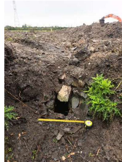
Plate 6: Field drain running into townland boundary ditch, facing south
