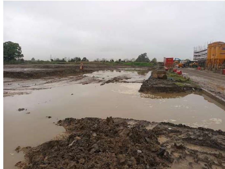
Plate 2: Northeast of development area, facing southwest
