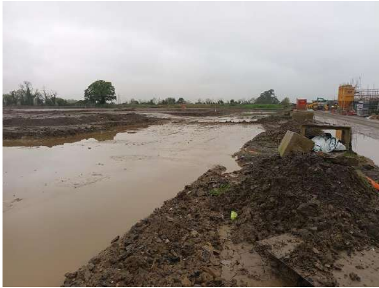
Plate 1: East-central of development area, facing west
