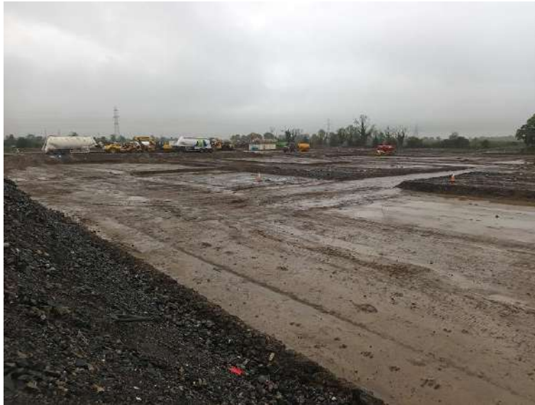
Plate 5: Subsoil of development area, facing southwest
