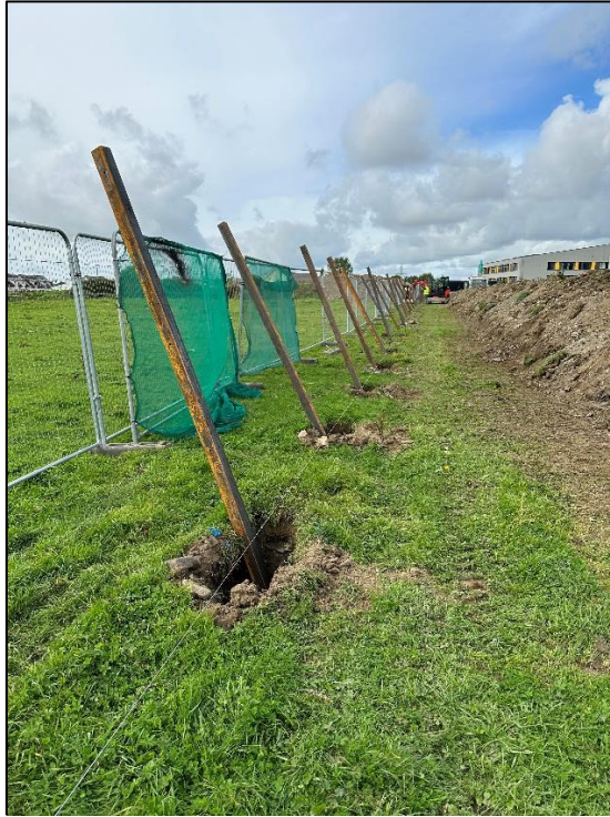
Plate 1 Investigation took place of excavated pits for fence posts
