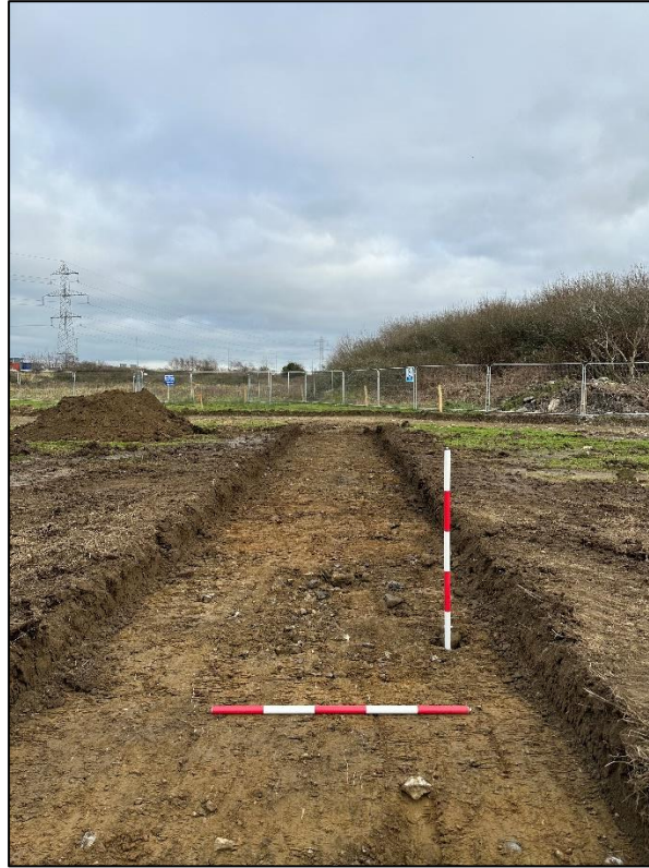
Plate 7 Stripping of topsoil for utilities and drainage
