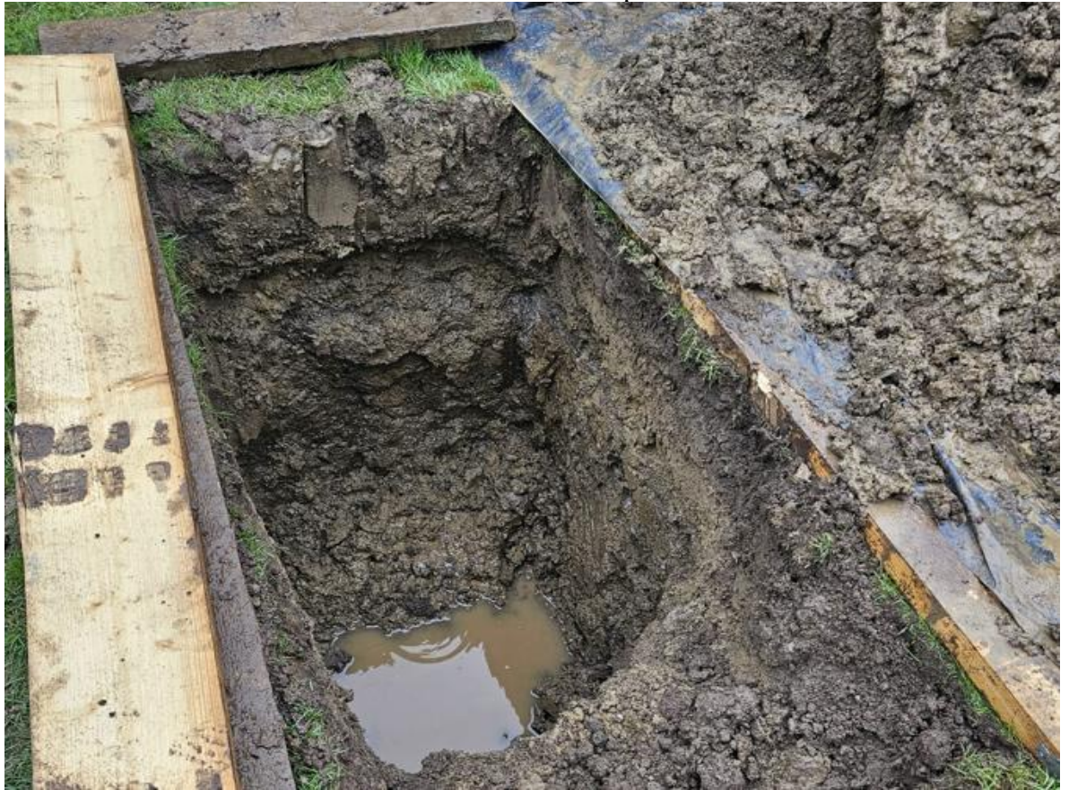
Photo Trial Pit after excavation – Depth 1.6
