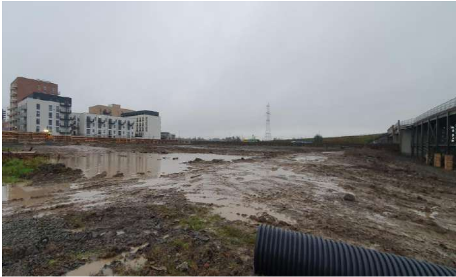
Plate 1: Southern portion of development area, facing southeast
