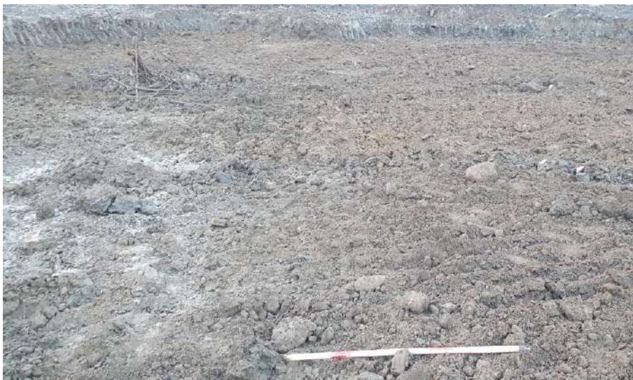
Plate 3: Disturbed ground (with buried metal rebar), facing north
