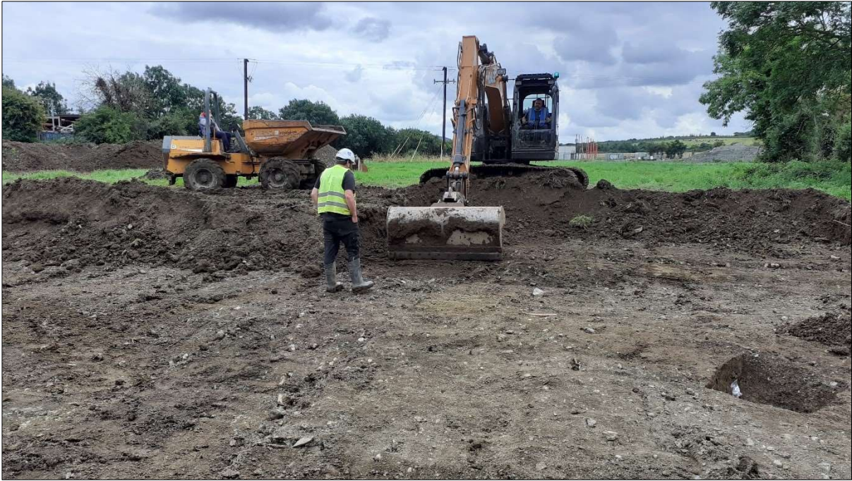
Plate 6: Working shot showing topsoil stripping, facing south
