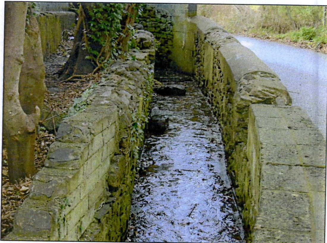
Photo 4: Stone Channel Upstream End
