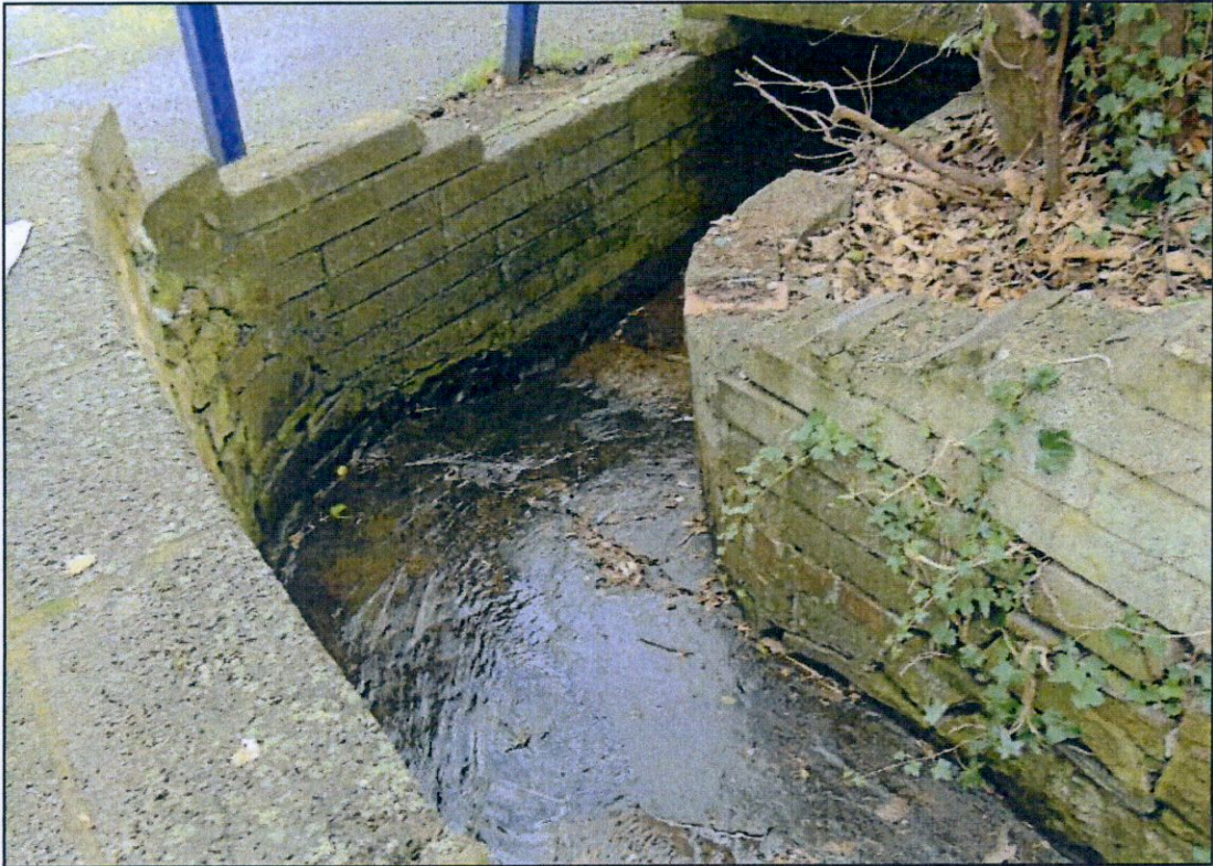
Photo 5: Stone Channel Downstream End
