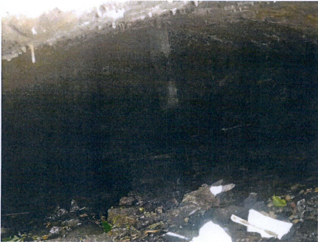
Photograph No. 3 Upstream End @ 2 m. Arch Barrel
