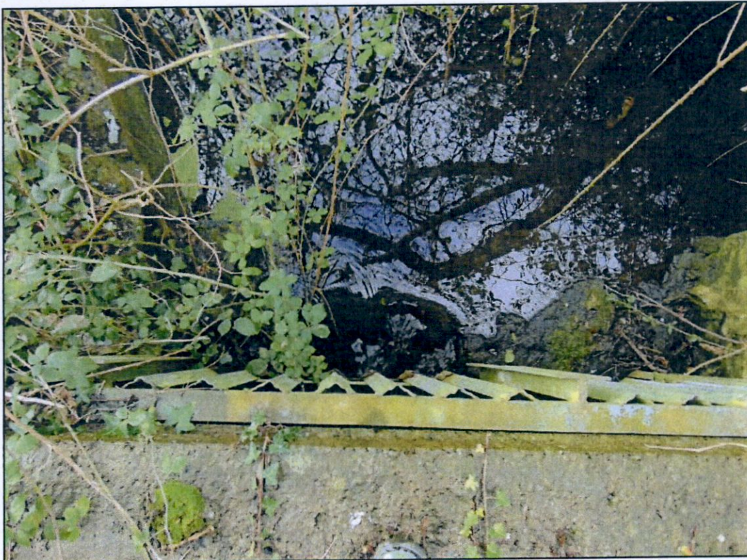
Photo 2: Pond Outlet into Concrete Tank
