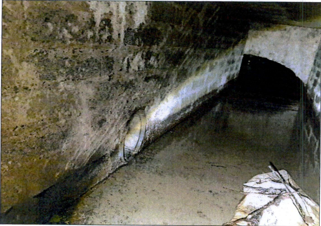
Photo 9: Stormwater Connection from Mill Pond Apartments
