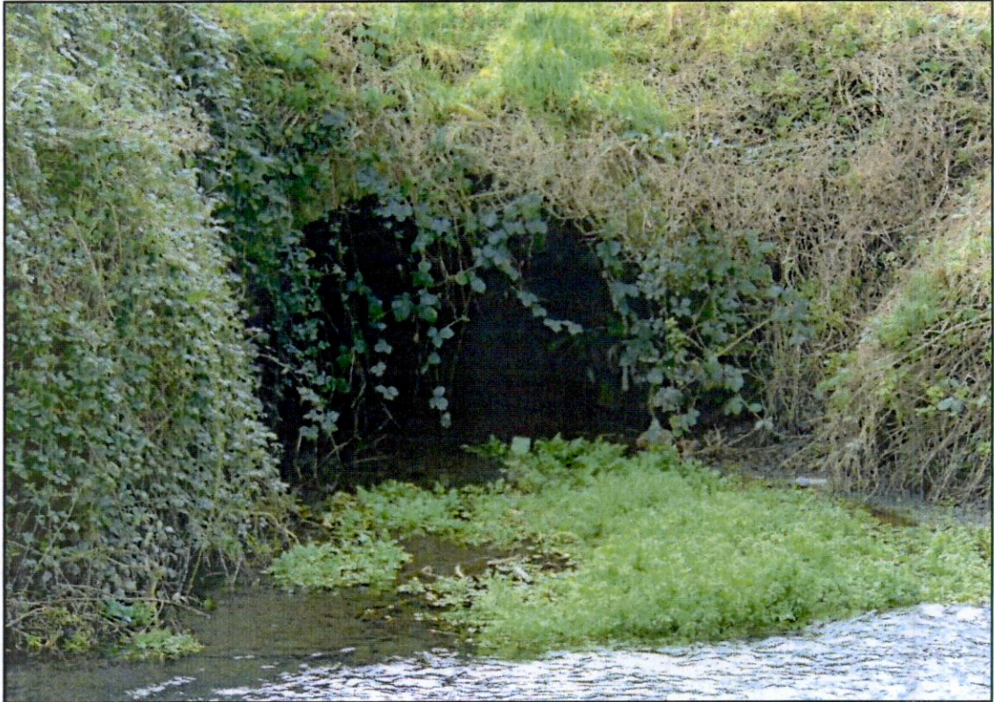
Figure 2 - Culvert Outlet to Camac River
