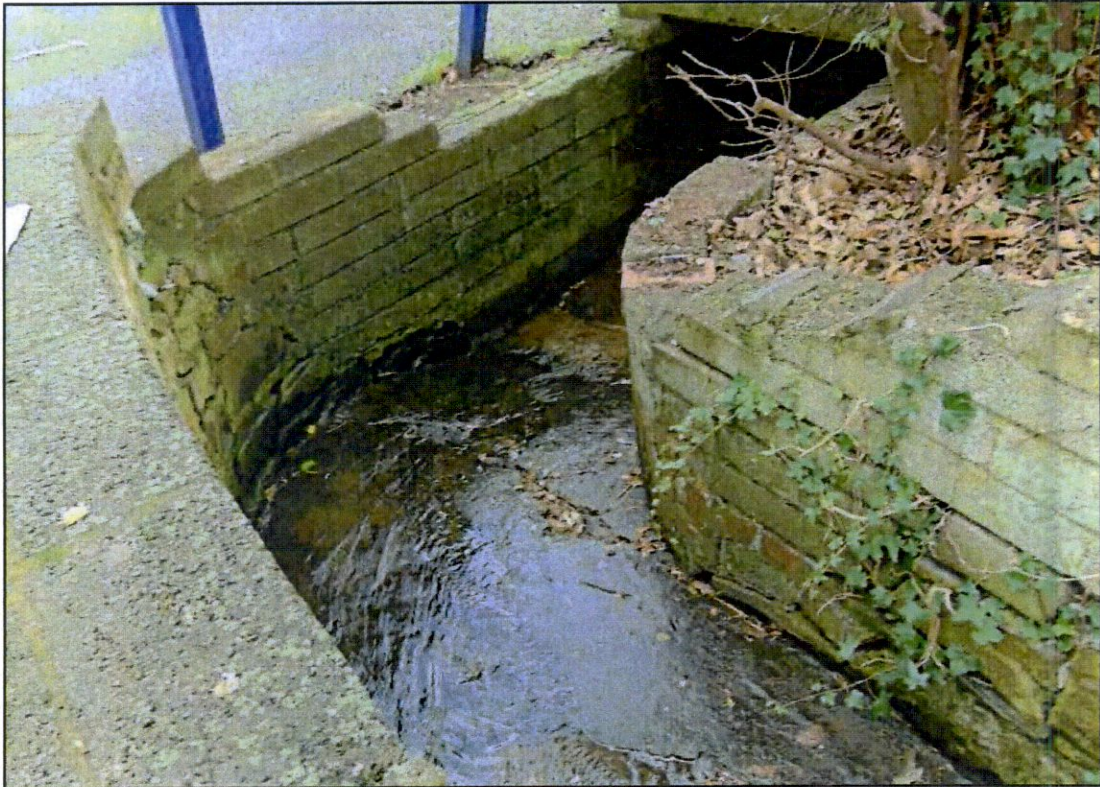
Photo 5: Stone Channel Downstream End
