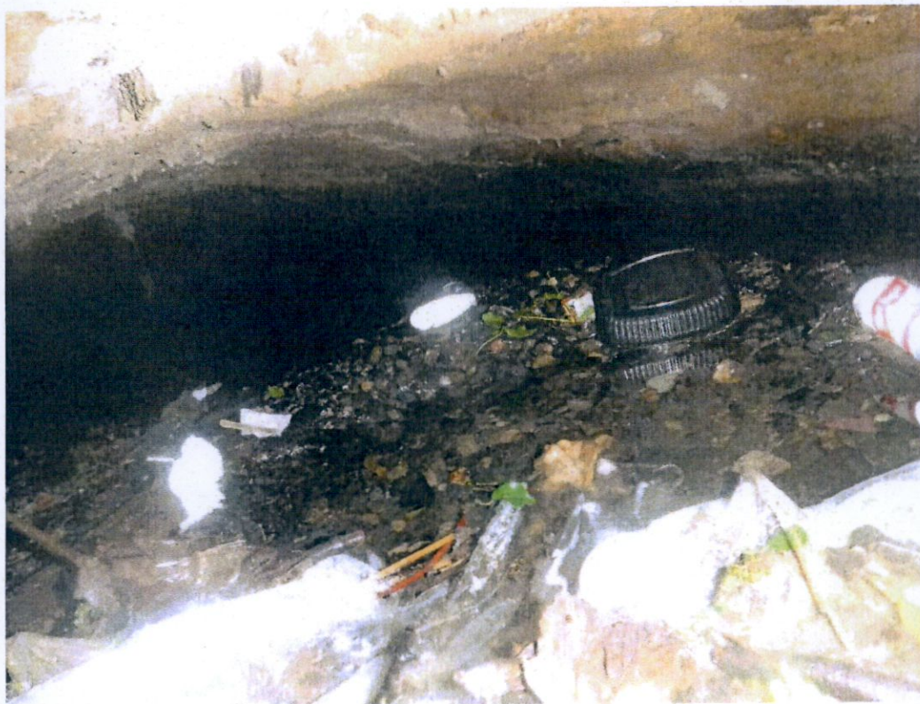
Photograph No. 4 Upstream End @ 2 m. Arch Barrel
