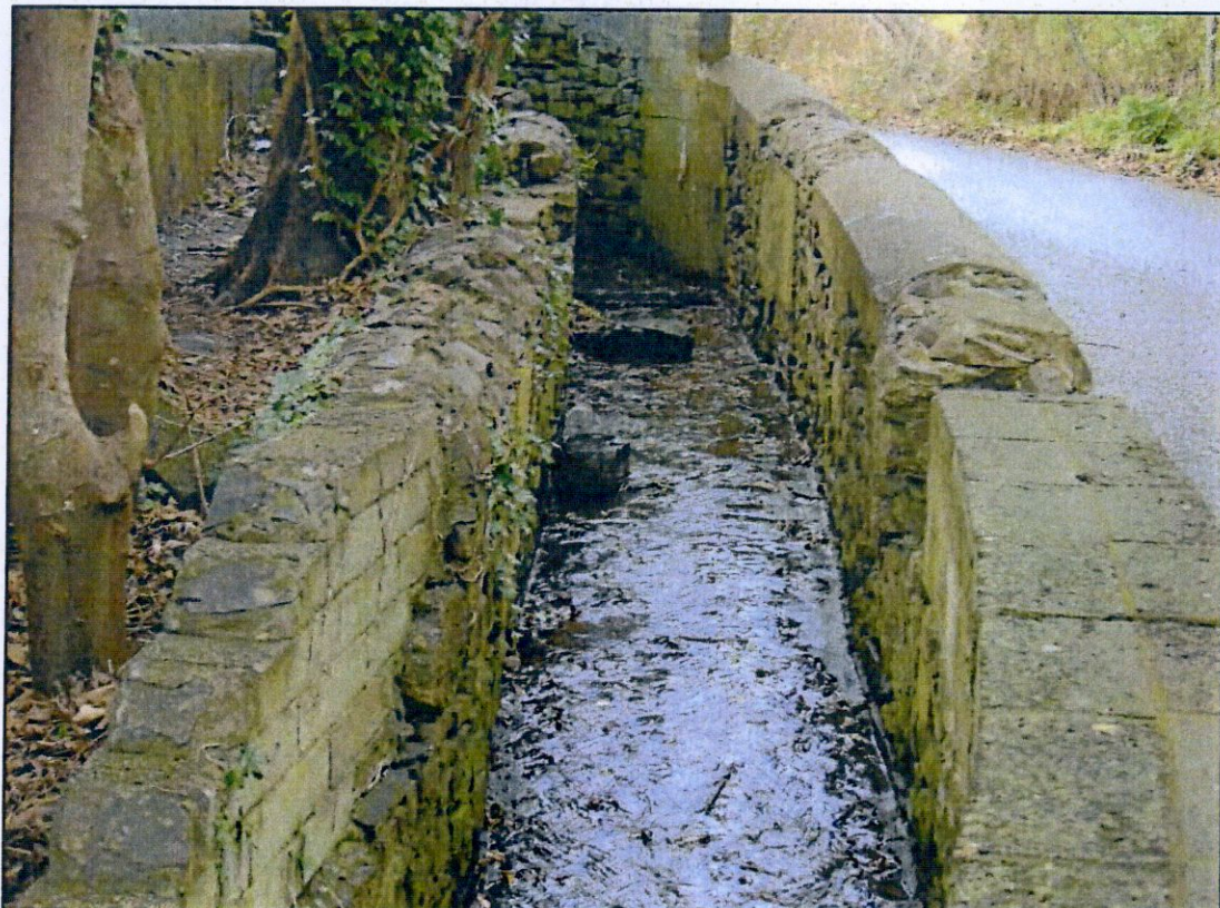
Photo 4: Stone Channel Upstream End
