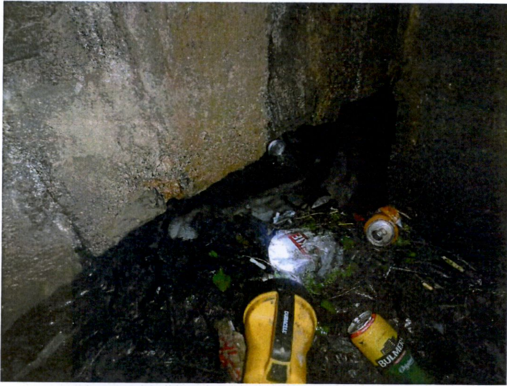
Photograph No. 1 Upstream end. Old bridge fascia.
