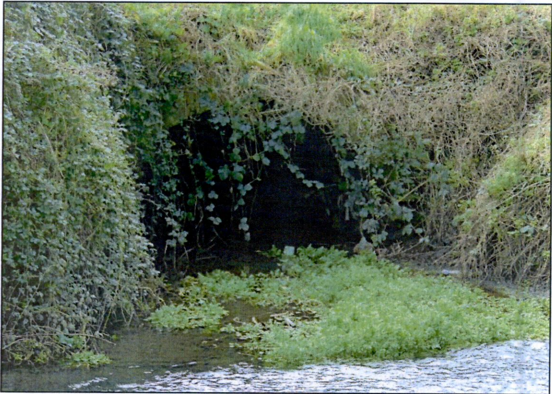
Photo 7: Culvert Outlet to Camac River
