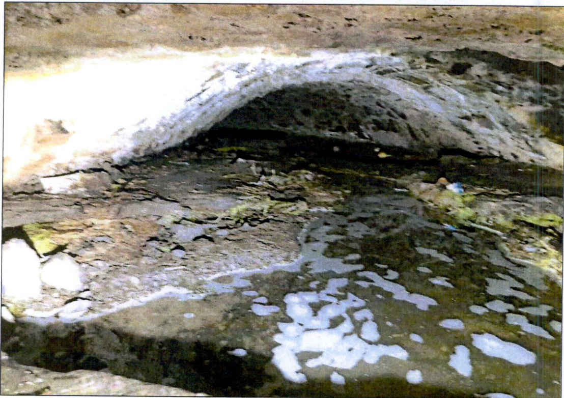
Photo 10: Culvert Looking Downstream from Rebuilt Section
