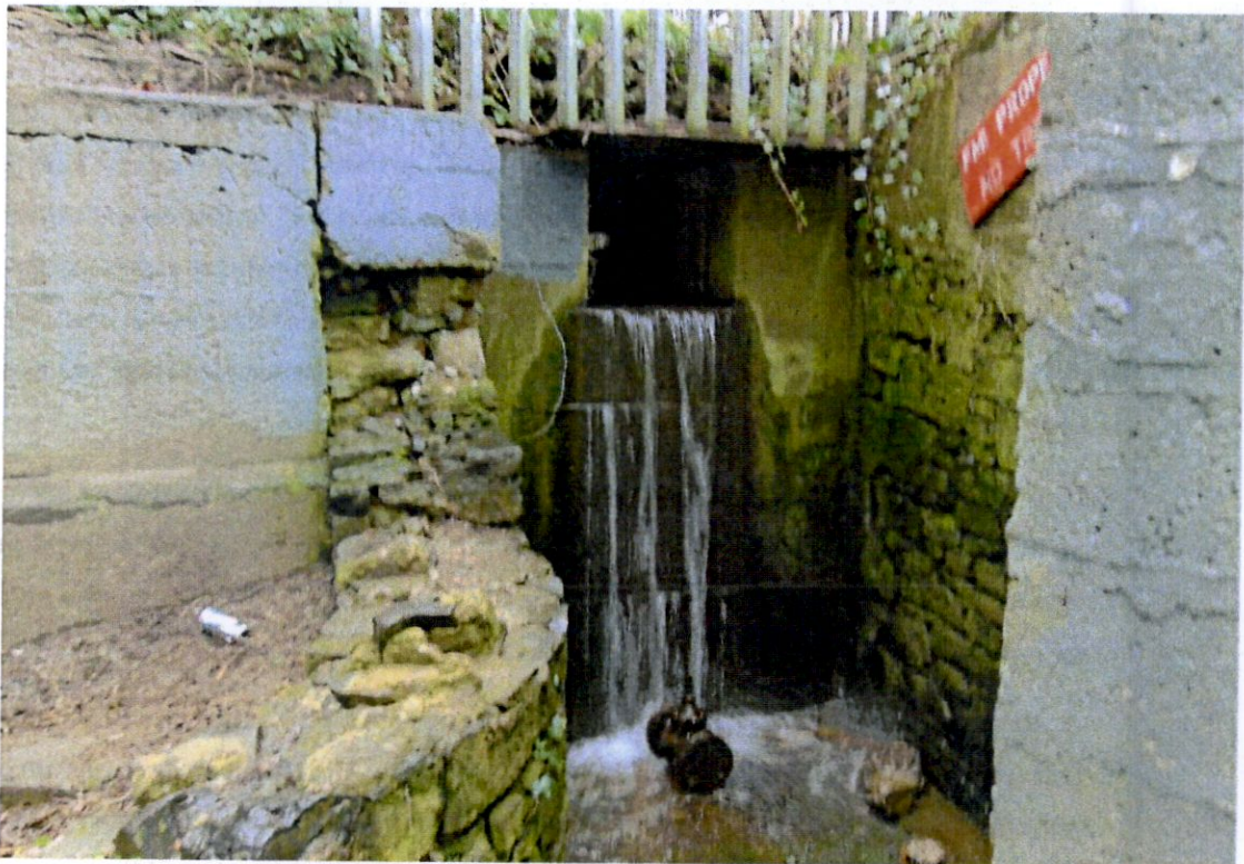
Figure 2 – Concrete Tank Outlet
