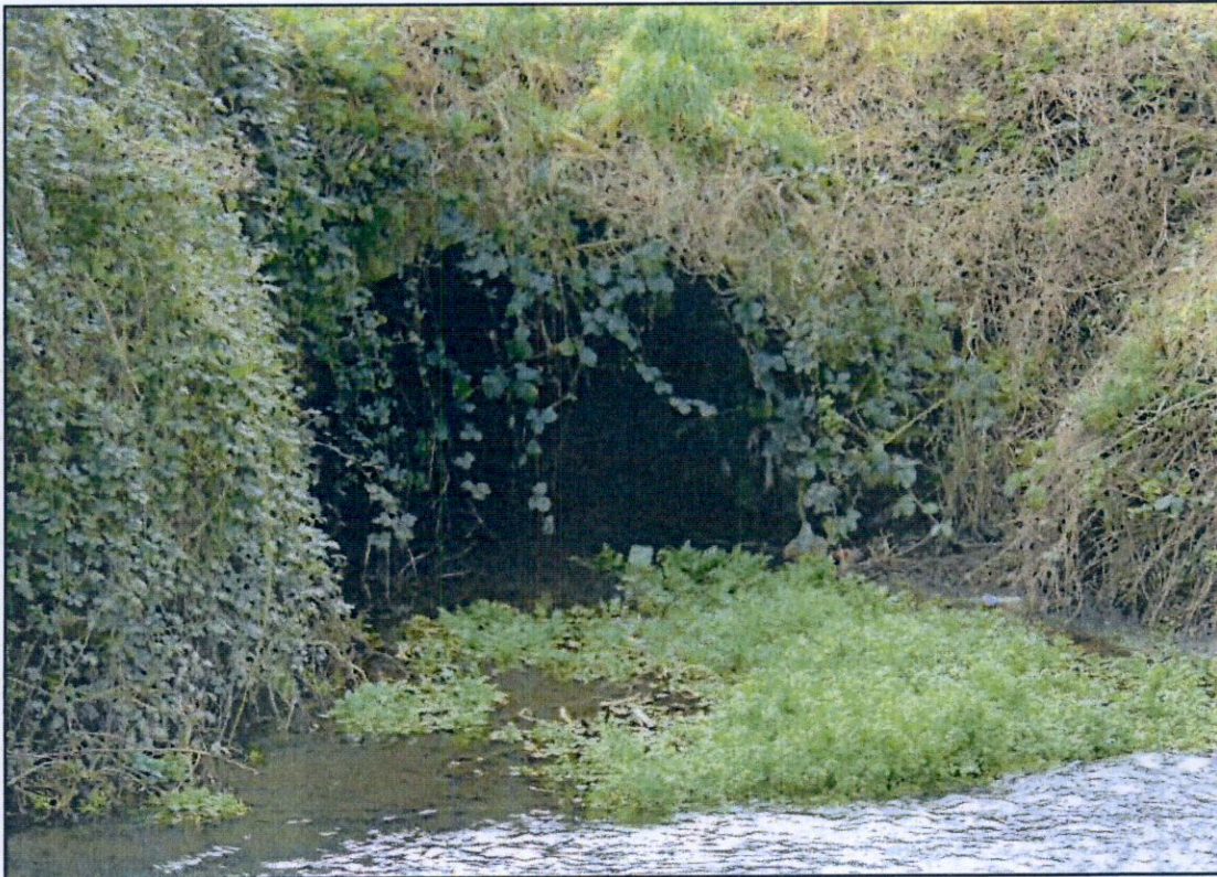
Photo 7: Culvert Outlet to Camac River
