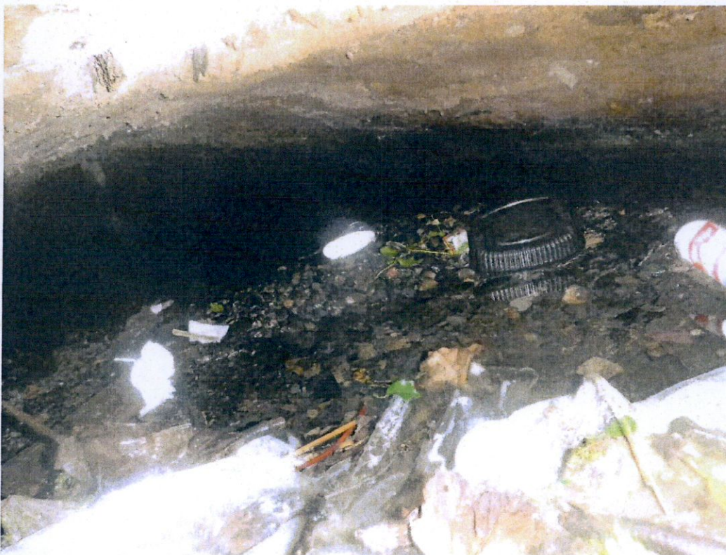
Photograph No. 4 Upstream End @ 2 m. Arch Barrel
