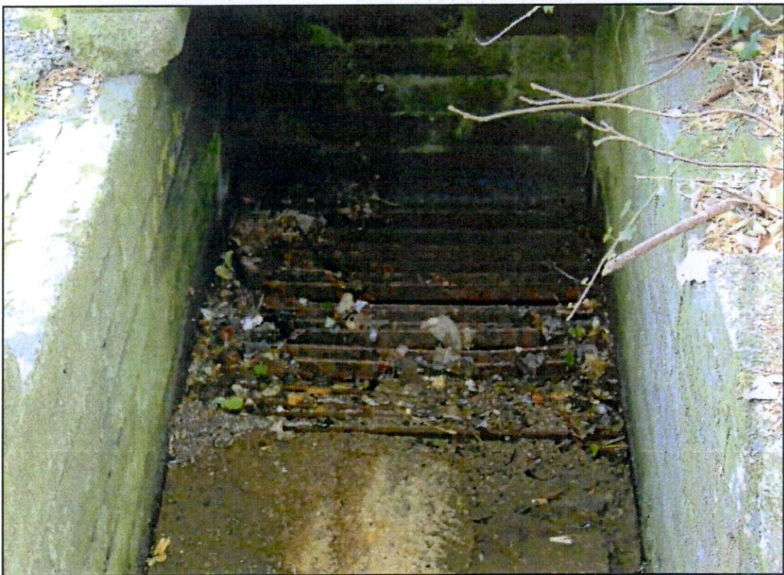
Photo 6: Sump Inlet & Grill
