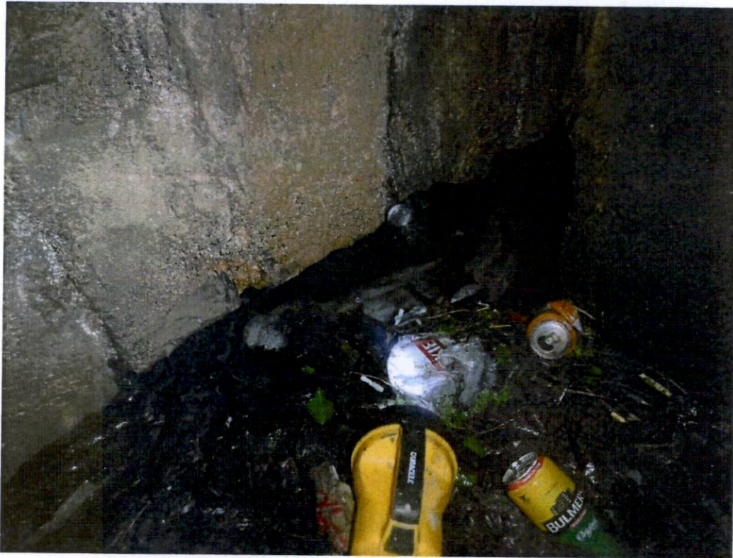
Photograph No. 1 Upstream end. Old bridge fascia.
