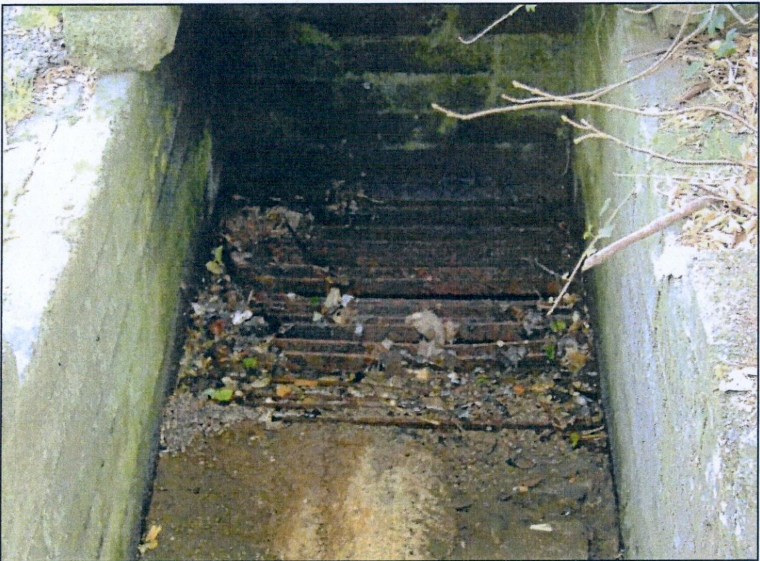
Photo 6: Sump Inlet & Grill
