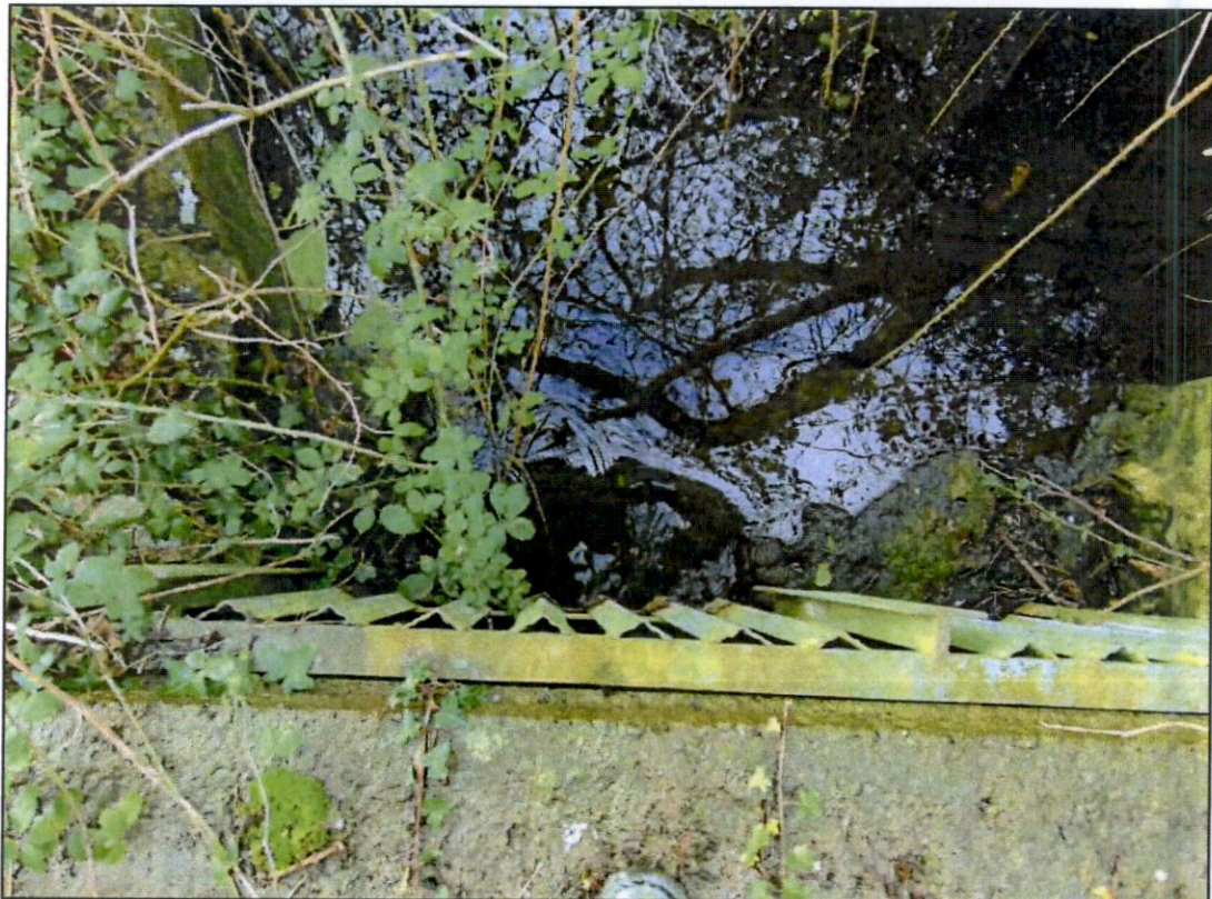
Photo 2: Pond Outlet into Concrete Tank
