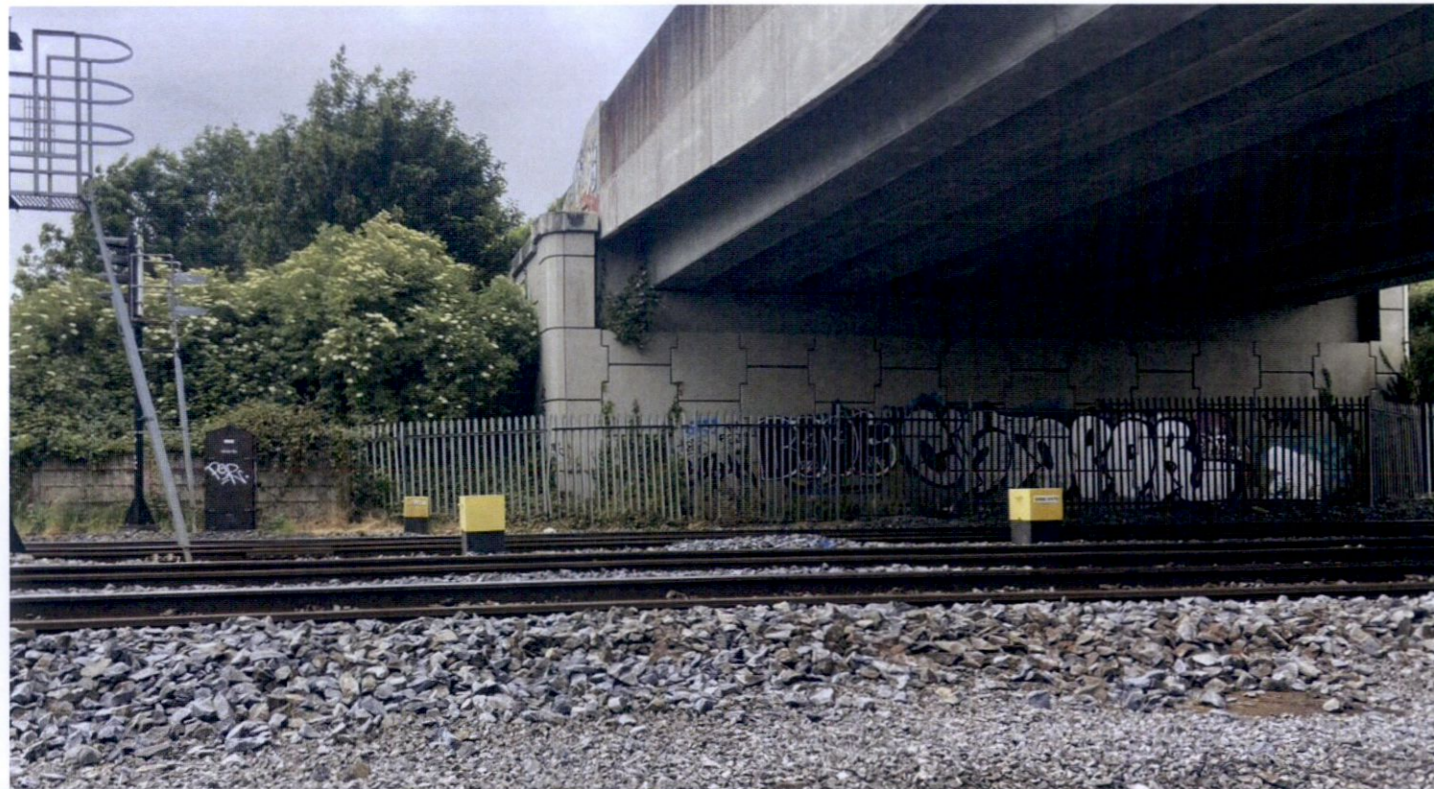
View beneath the R120 railway overbridge showing the southern abutment and north-west corner of the site.
