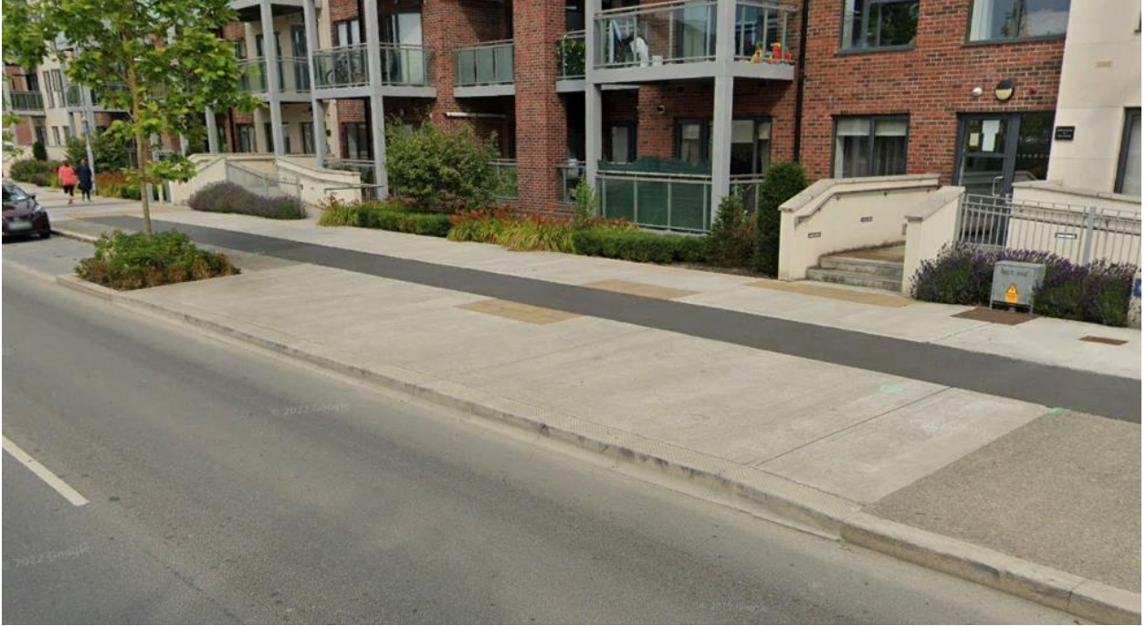
Figure 4: Existing bus stop with segregated footpath and cycle track on Shackleton Drive, Adamstown
