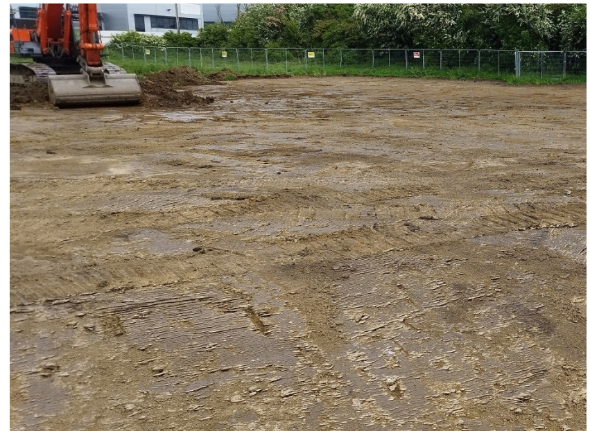
Plate 8: General view, north extent, looking northwest.
