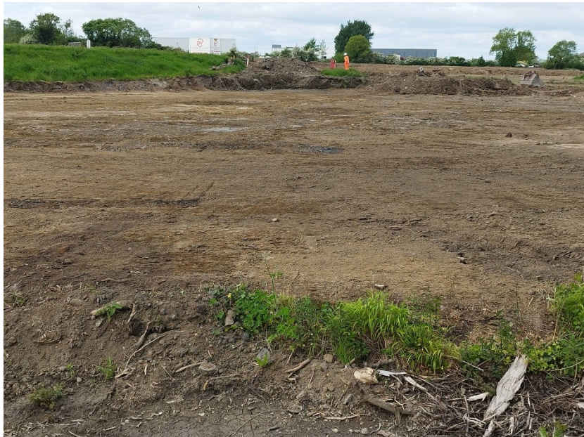
Plate 15: General view, looking northwest.
