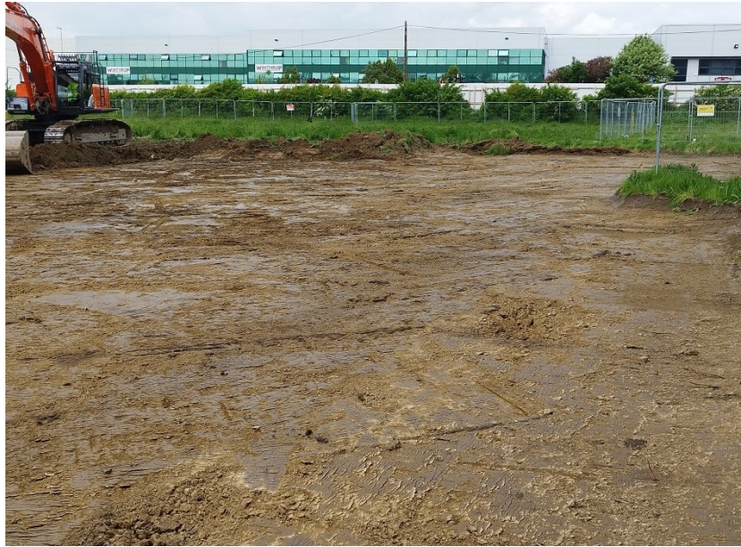
Plate 13: General view, north end, looking north.
