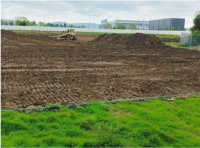
Plate 1: General view, looking southwest.
