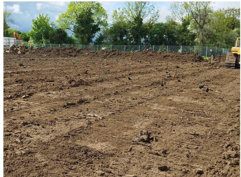
Plate 4: General view, looking northwest.
