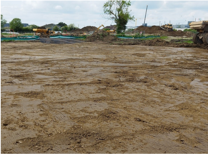
Plate 5: General view, northeast extent, looking northwest.
