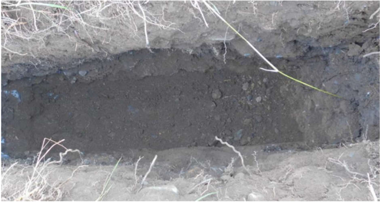
Trial Pit 1.5m deep no water table
