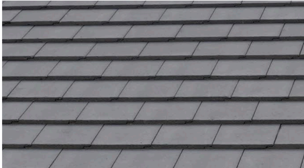
ROOF FINISH 01 (CONCRETE TILE) - RF01
