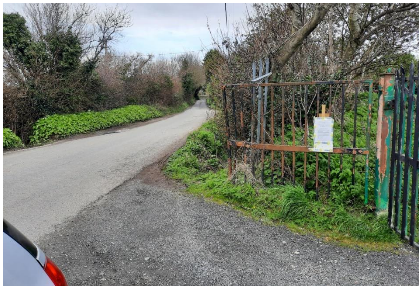
Picture showing fencing panel obscuring sight line for vehicles leaving
