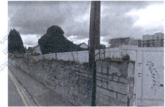
Existing site entrance and stone wall boundary
