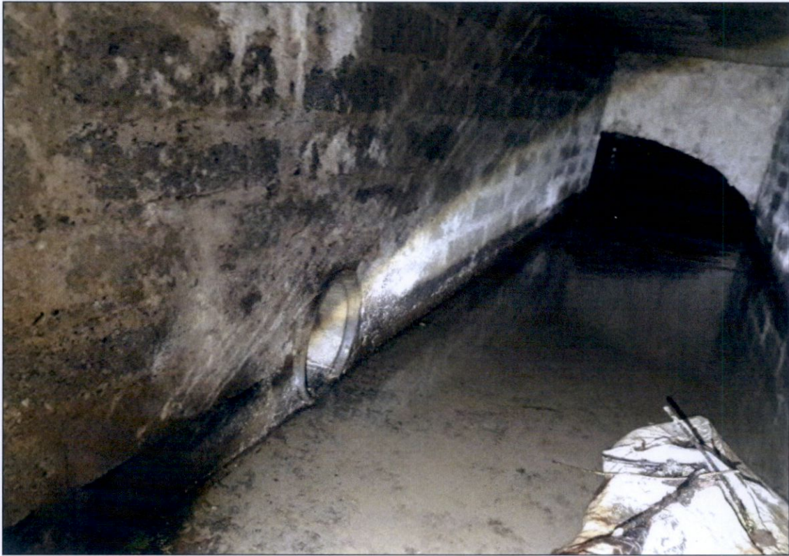
Photo 9: Stormwater Connection from Mill Pond Apartments
