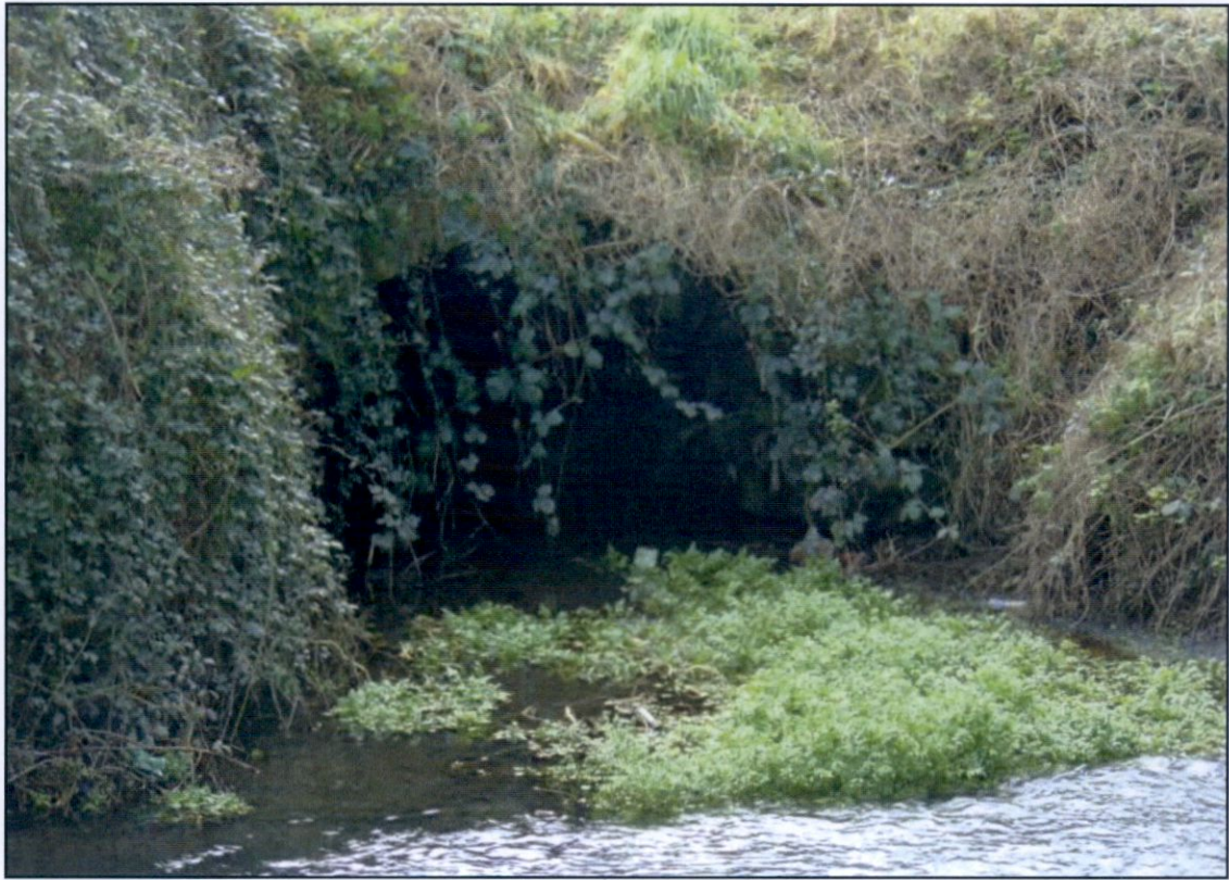
Photo 7: Culvert Outlet to Camac River
