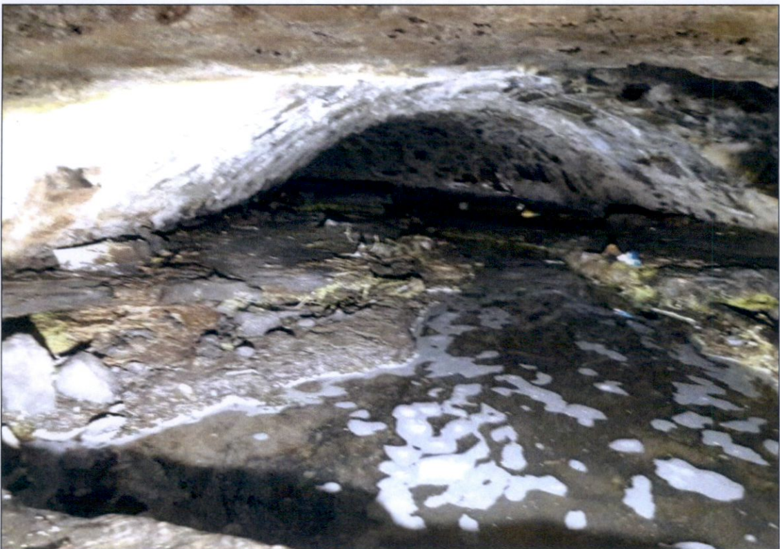
Photo 10: Culvert Looking Downstream from Rebuilt Section
