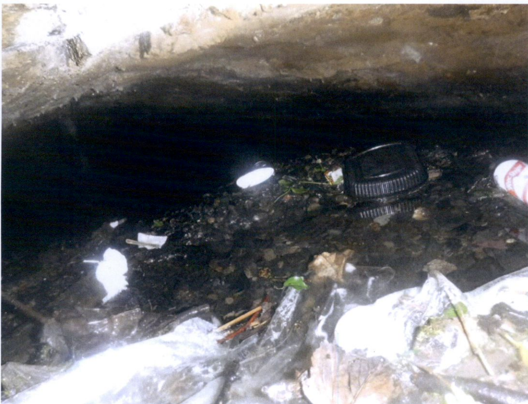
Photograph No. 4 Upstream End @ 2 m. Arch Barrel
