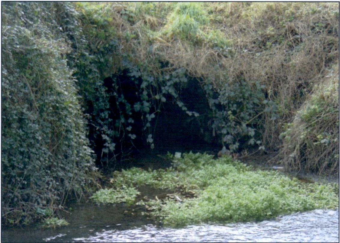
Figure 2 - Culvert Outlet to Camac River
