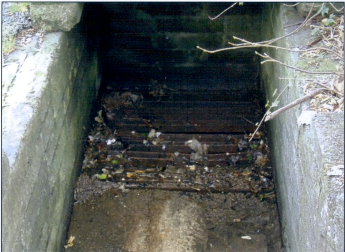
Photo 6: Sump Inlet & Grill
