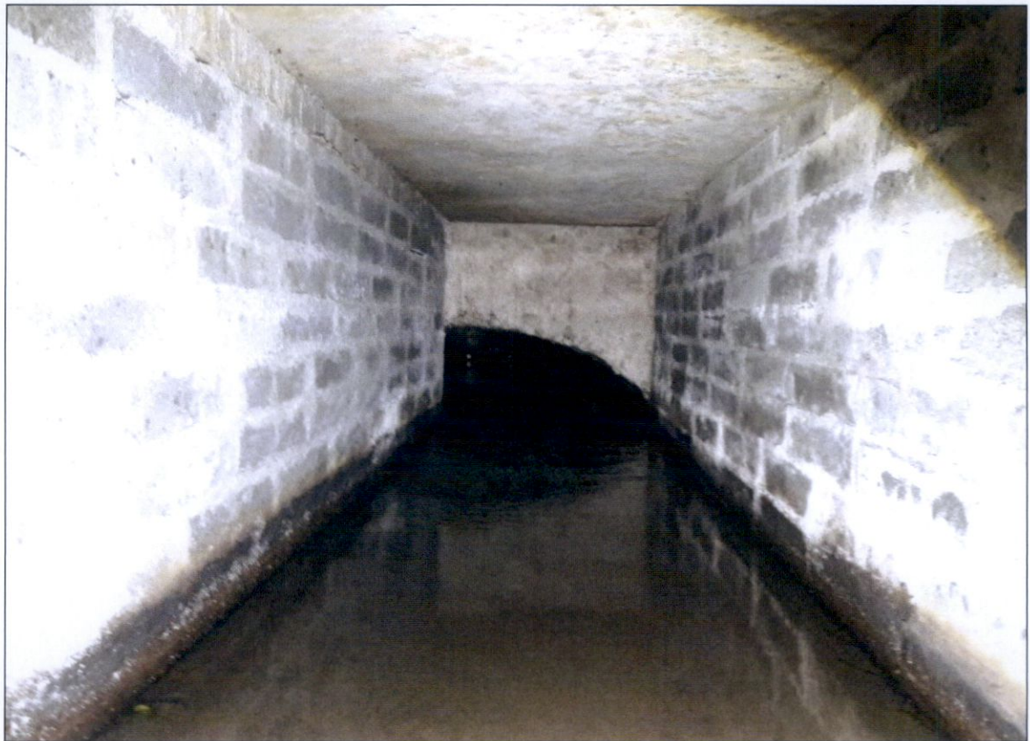
Photo 8: Rebuilt Culvert Outside Mill Pond Apartments Looking Upstream
