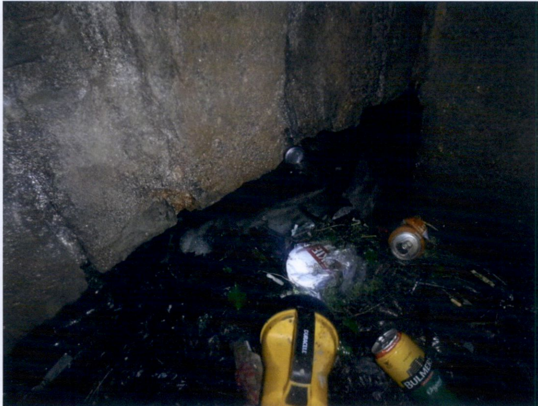
Photograph No. 1 Upstream end. Old bridge fascia.
