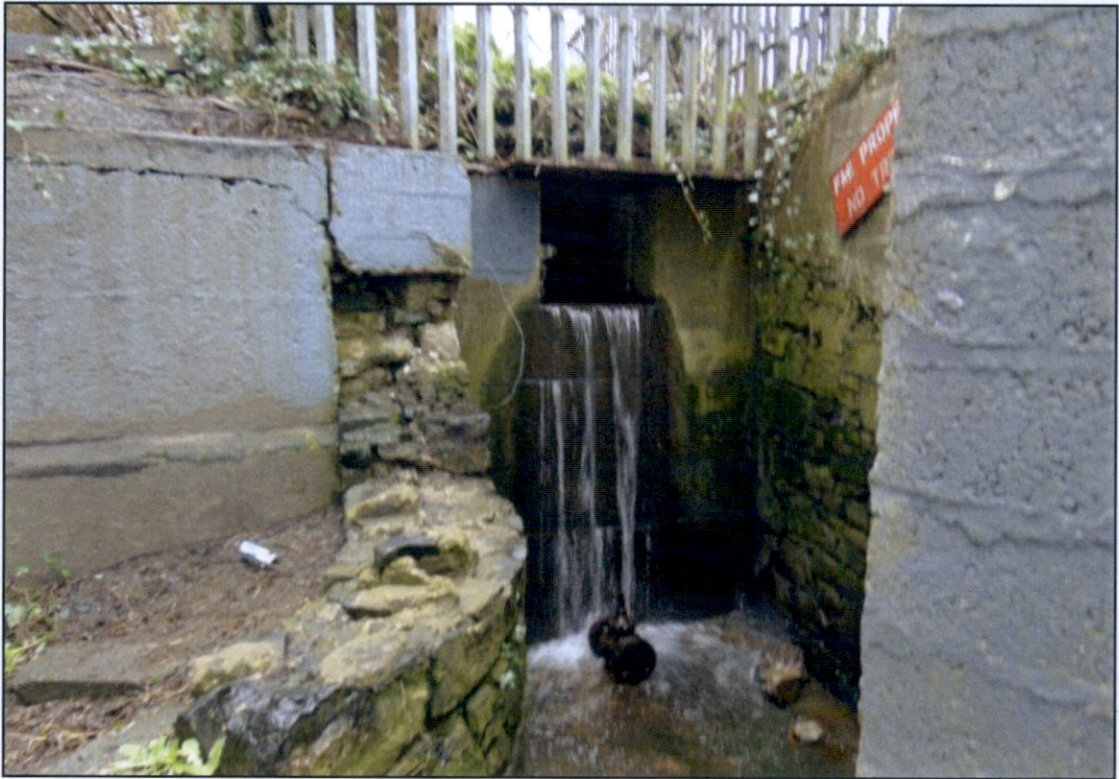
Figure 3 – Concrete Tank Outlet
