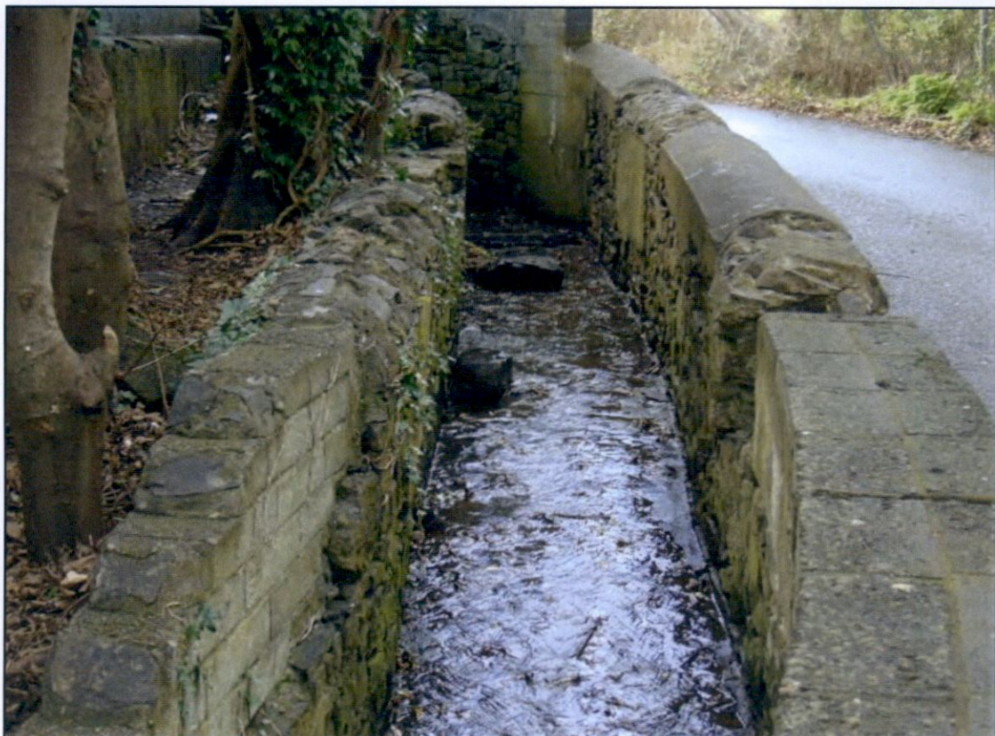
Photo 4: Stone Channel Upstream End
