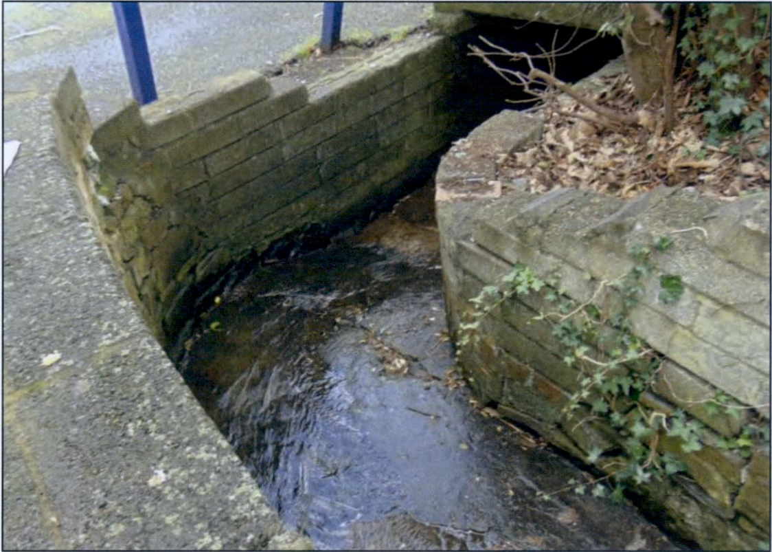
Photo 5: Stone Channel Downstream End
