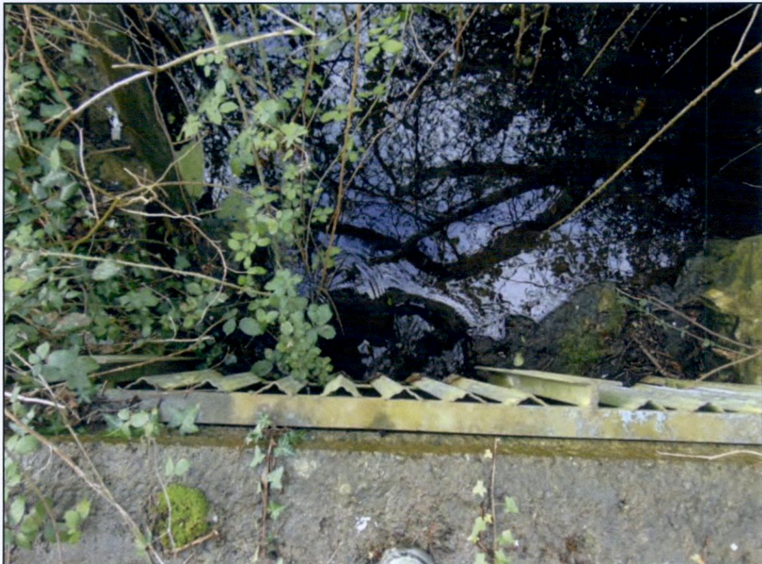
Photo 2: Pond Outlet into Concrete Tank
