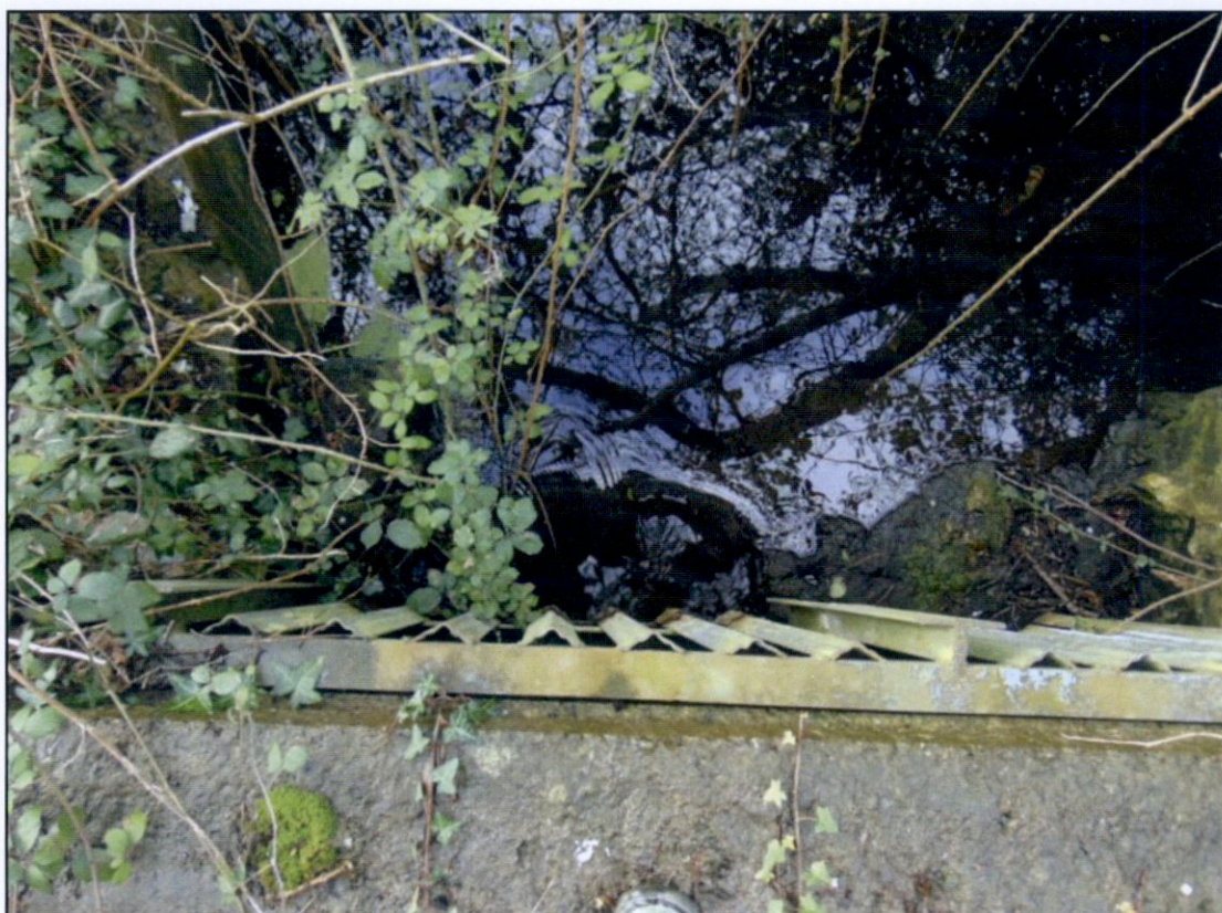
Photo 2: Pond Outlet into Concrete Tank
