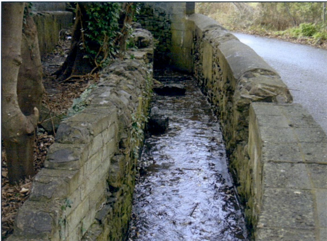
Photo 4: Stone Channel Upstream End
