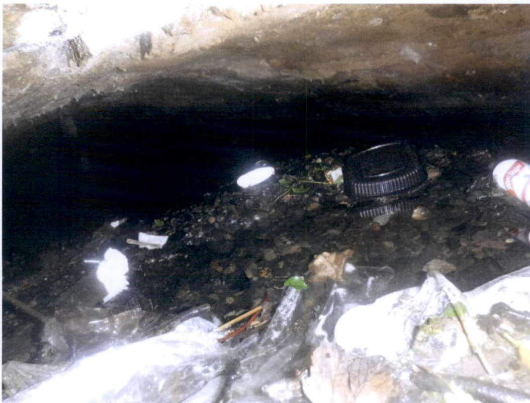
Photograph No. 4 Upstream End @ 2 m. Arch Barrel
