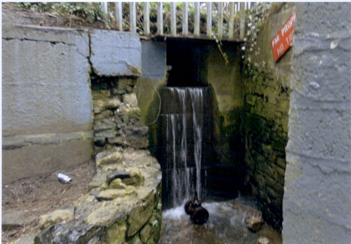
Figure 2 – Concrete Tank Outlet
