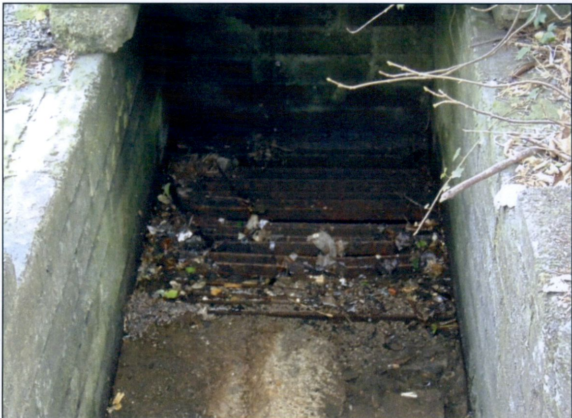
Photo 6: Sump Inlet & Grill
