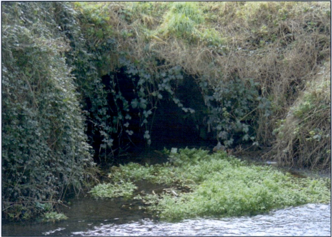
Photo 7: Culvert Outlet to Camac River
