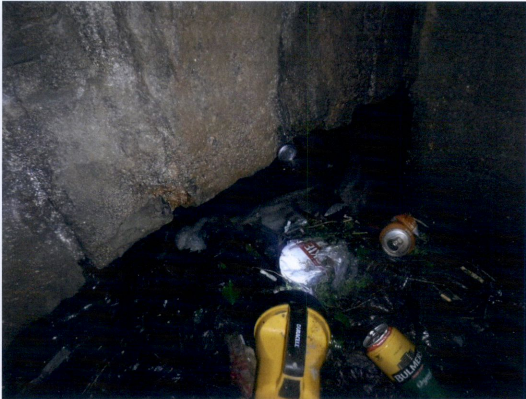
Photograph No. 1 Upstream end. Old bridge fascia.
