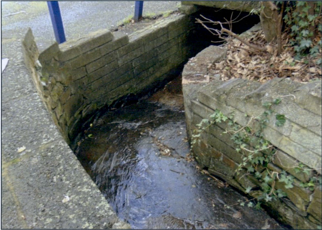
Photo 5: Stone Channel Downstream End
