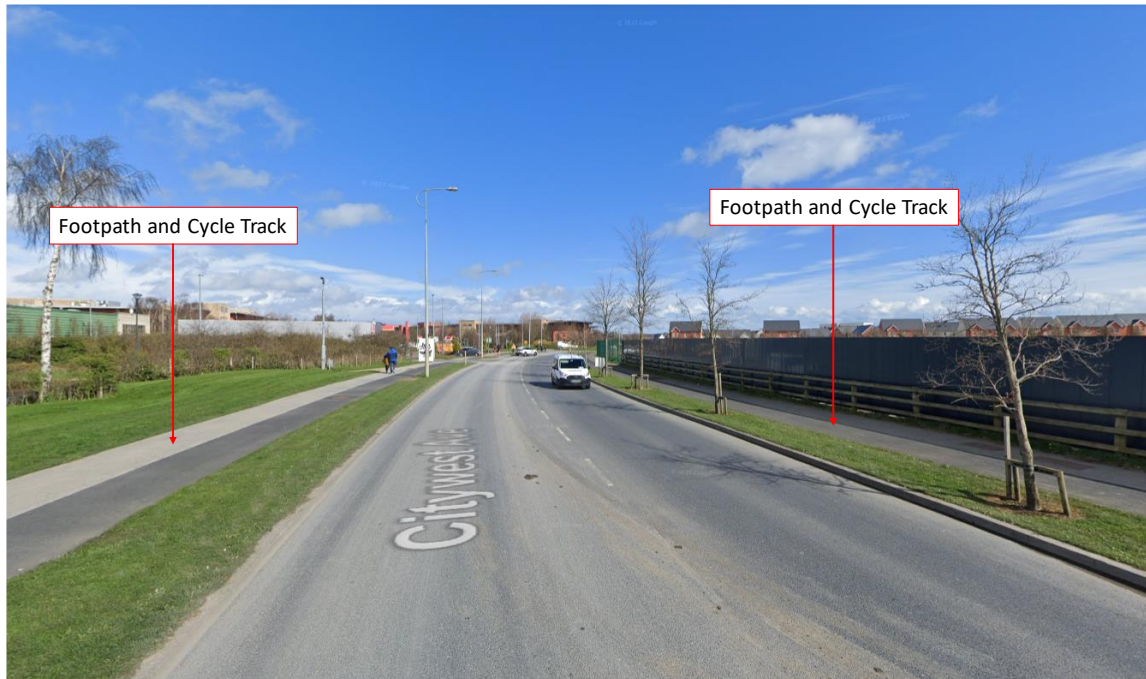
Figure 2.2 – Cycle Facilities on Citywest Avenue
