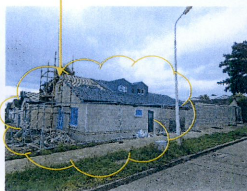
As built west view.
