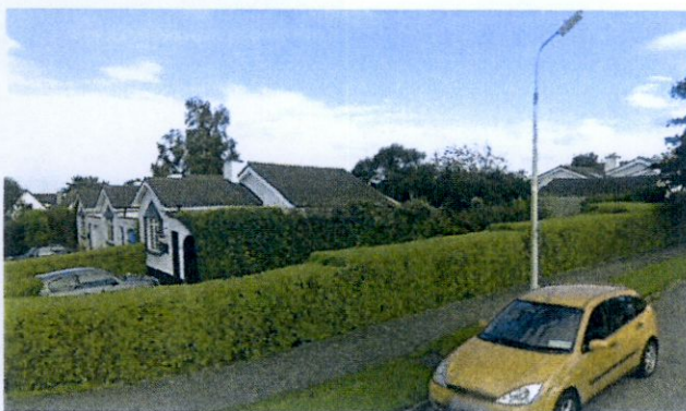
Original west view.
