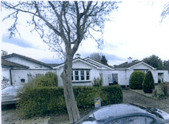
Original front view.
