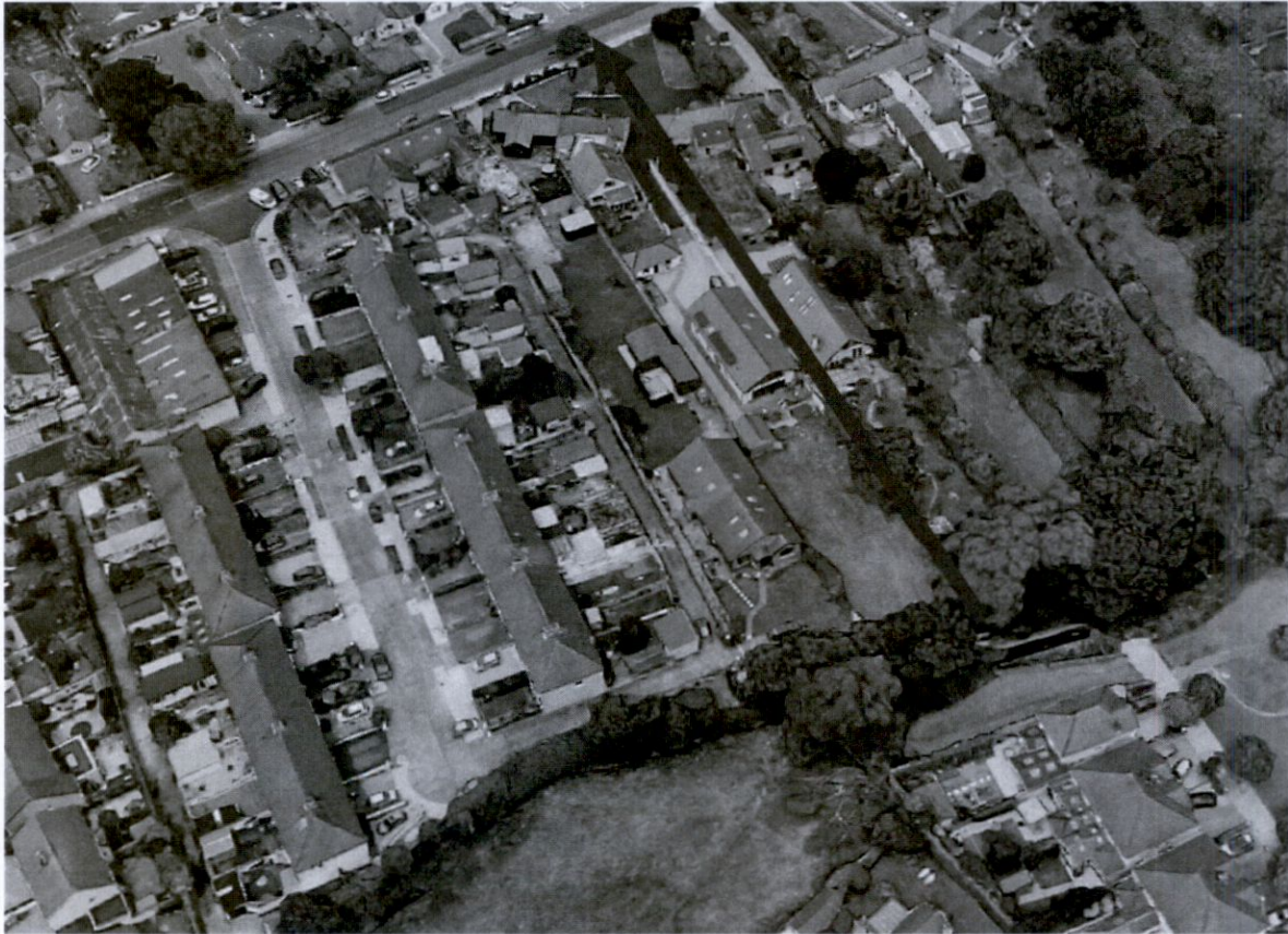
Figure 12 Pathway of the Source Receptor Flood Water Onto Whitehall Road
