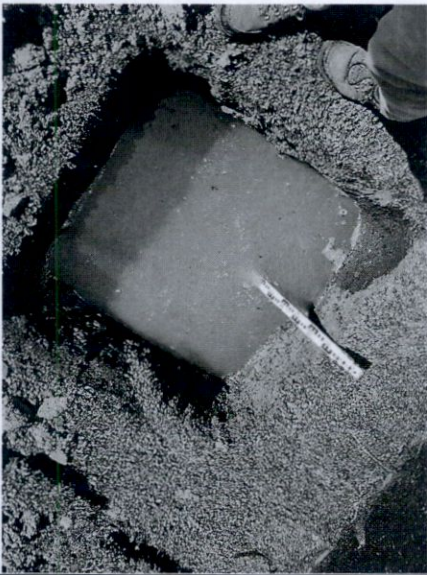
Soakaway Under Test
