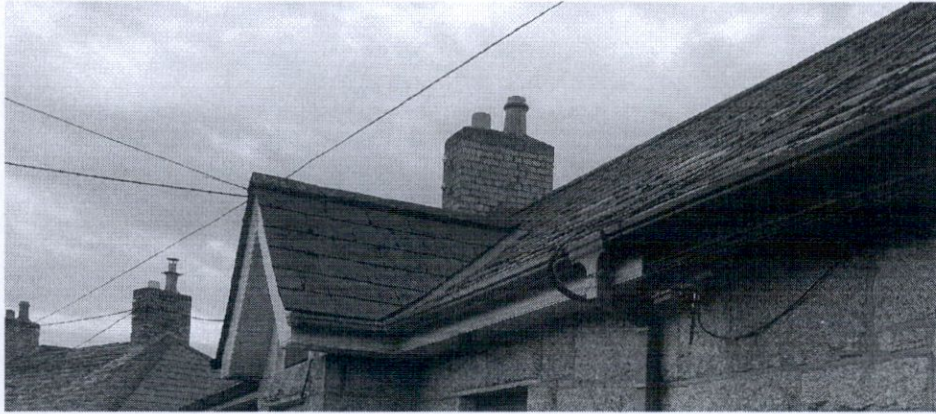
Brick chimney on 184, 186 have been rendered.
