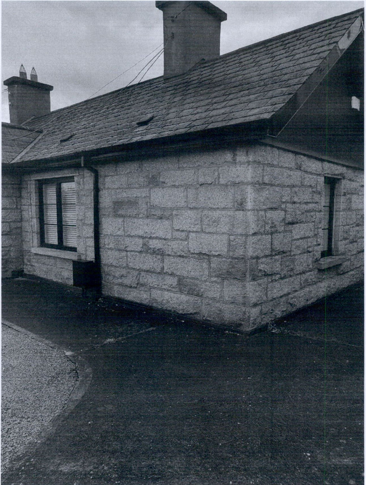
Pitched roof style at 186, note slates are not original
