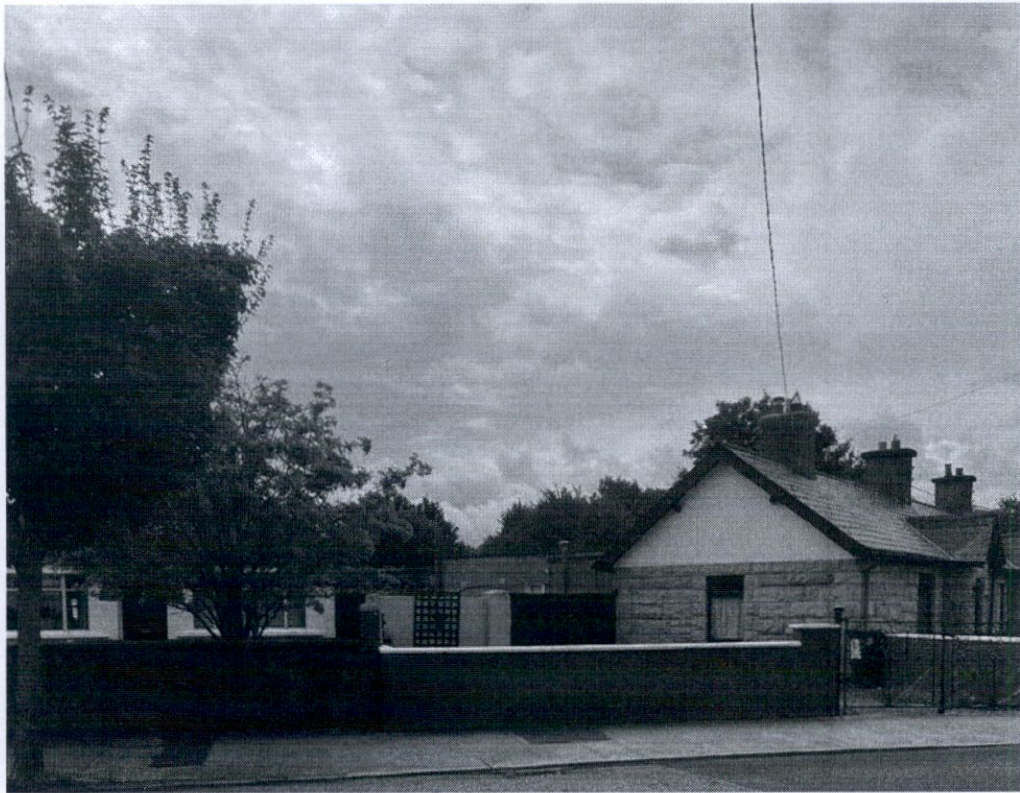
168 Whitehall Road has a single storey extension visible at street level
