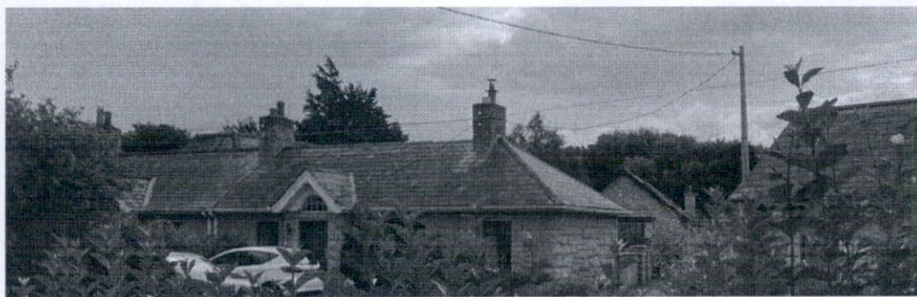
The dwelling built in the rear of 182 is visible as is the extension directly joining the cottage at 180
