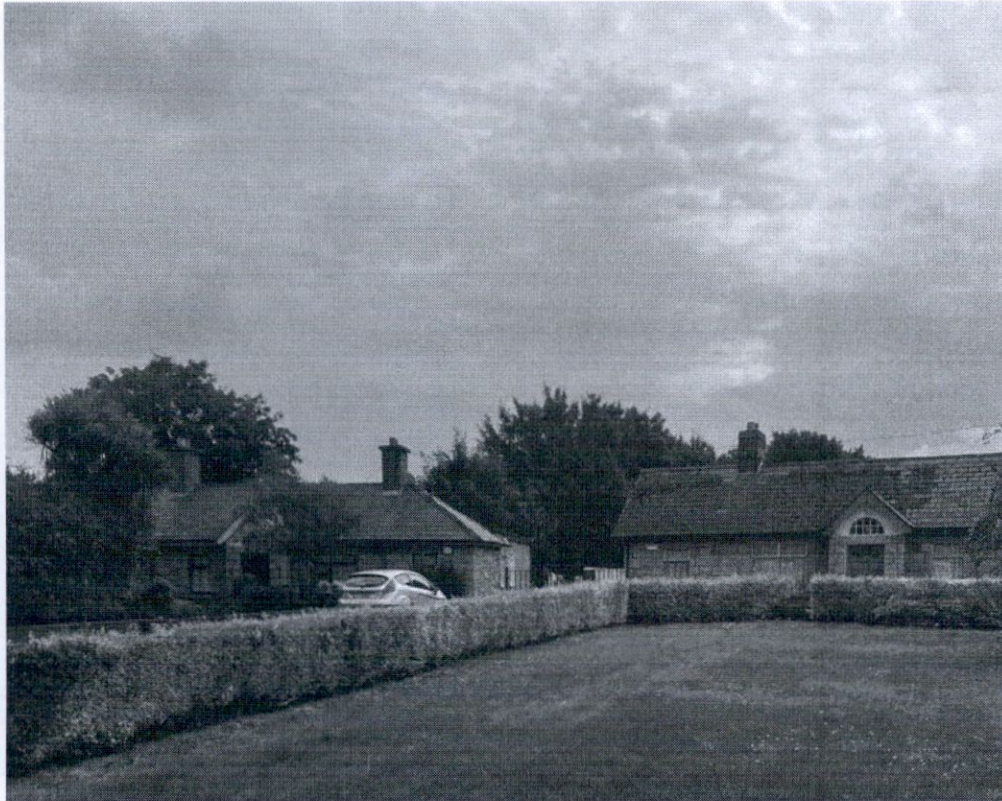
176 Whitehall Road has a single storey extension that abuts the cottage directly and in no way compliments or enhances the architectural features of the cottage, it is also visible from the street.
