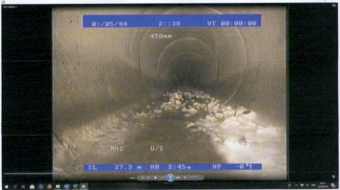
Debris & standing water. No connections
