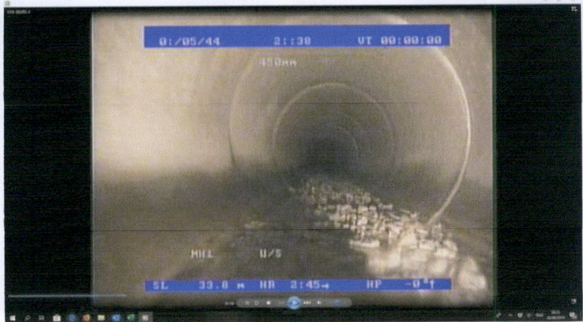
Debris in pipe. No connections
