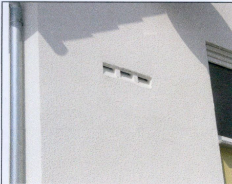
Figure 14. 3 no. combined bat brick tubes ('2FR' multiple bat tubes by Schwegler), refer to architect's drawings of elevations for exact locations
