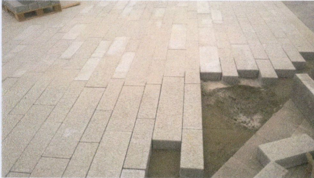
Figure 4. Pre-cast concrete unit paving, laid with proprietary spacers
