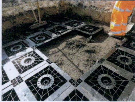
Figure 11. 'Arborflow' by GreenBlue Urban SuDS tree pit, filled with bio-retention type soils
