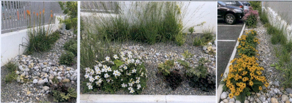
Figure 13. Images of simple rain garden strip in a car park, south county Dublin. Check-dam, gravel mulch and moisture-tolerant perennial planting shown
