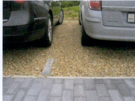
Figure 5. 'Nidagravel' grid filled with angular gravel
