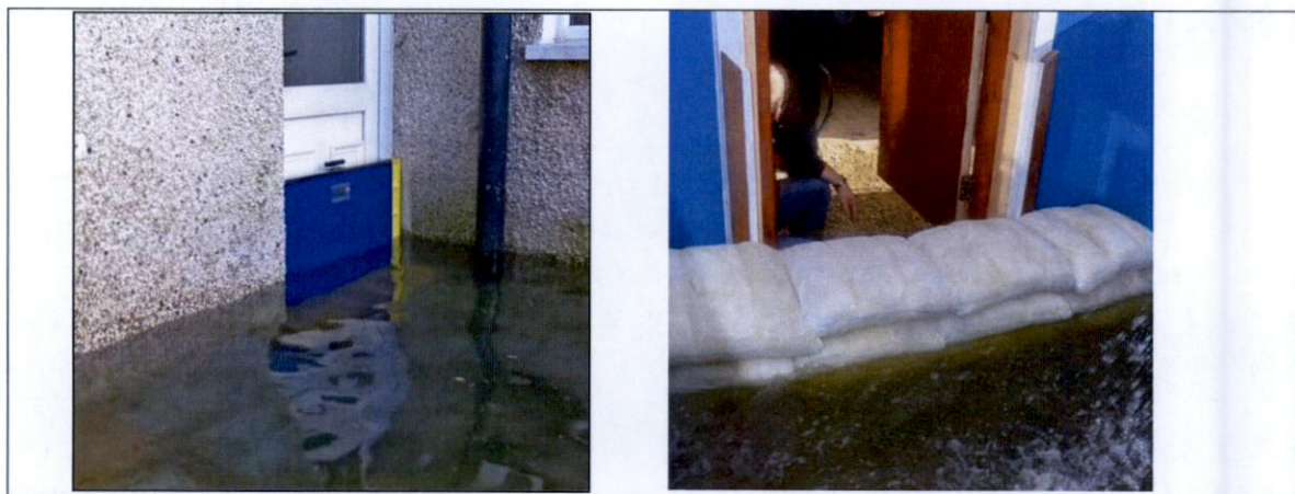
Plate 4 Flood Resilience measures: De-mountable 'Dam Easy barrier' and 'Flood Guard' synthetic sandbags (stackable to 1metre)
