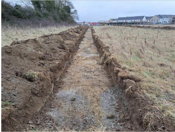
Plate 5: Test Trench 1, facing northeast
