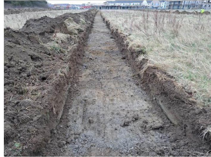
Plate 6: Test Trench 2, facing northeast
