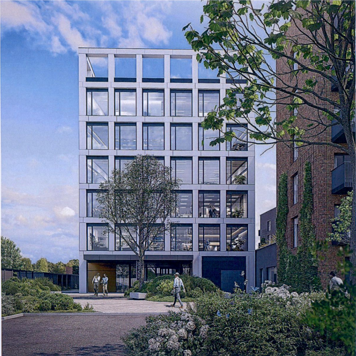
Illustration of Landmark building public realm, eastern area (computer generated image prepared by 3DDB)
