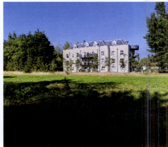
Figure 11 - View of existing structures in the western boundary (Residential)
