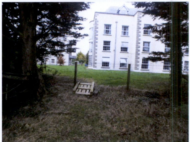
Plate 3. Apartments located just to east of the site.
