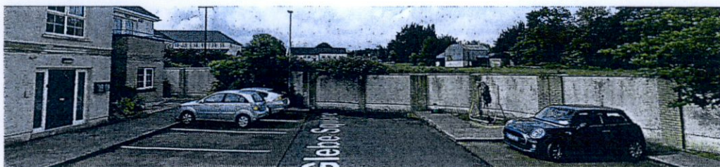
Boundary Wall at end of Road 4 Glebe Square.
