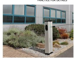
TYPICAL GARO TYPE (OR EQUAL AND APPROVED) 2nr CAR CHARGING STATION TO BE PART M COMPLIANT
