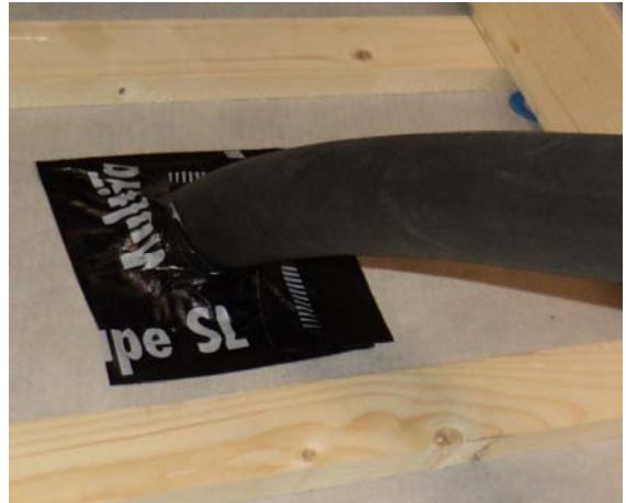
Figure 10: Sealing of Roof Underlay
