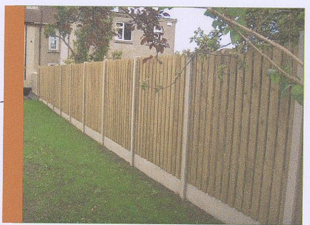
1.8m high Concrete Post and Timber Panel Fence Boundary Type 3
