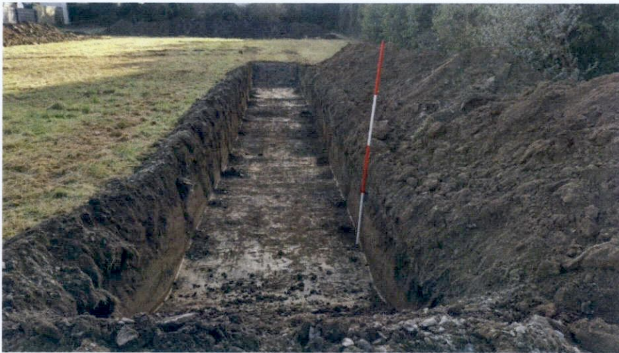
Plate 5 Trench 4 from the north
