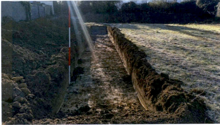
Plate 7 Trench 5 from the north
