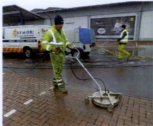
Figure 20.30 Deep cleaning a supermarket car park, Dundee (courtesy Abertay University)
