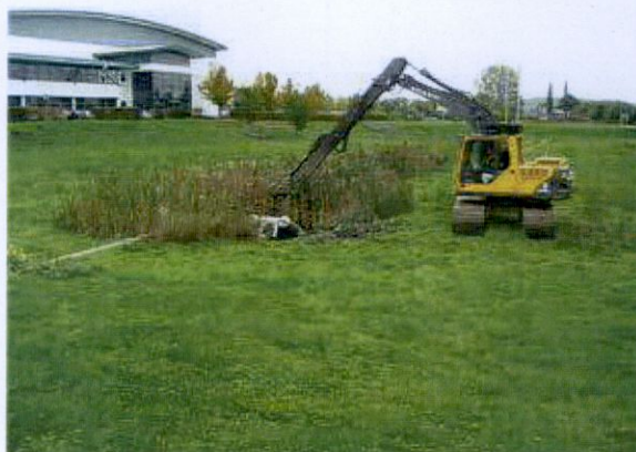
Figure 32.2 De-silting (courtesy Bedford Group of Drainage Boards)
