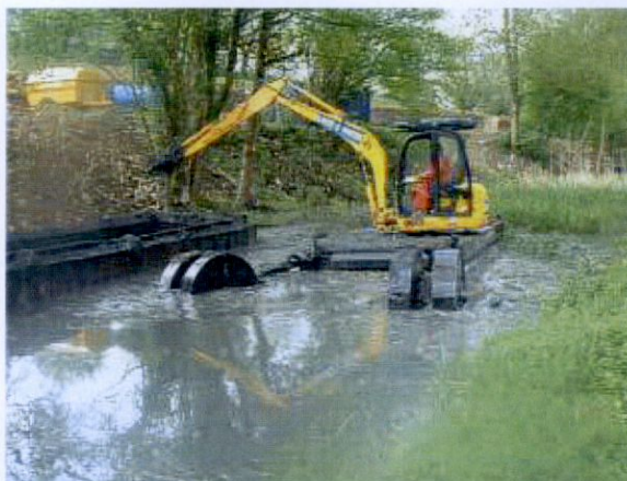
Figure 32.3 Floating excavator working in small pond (courtesy Land & Water)
