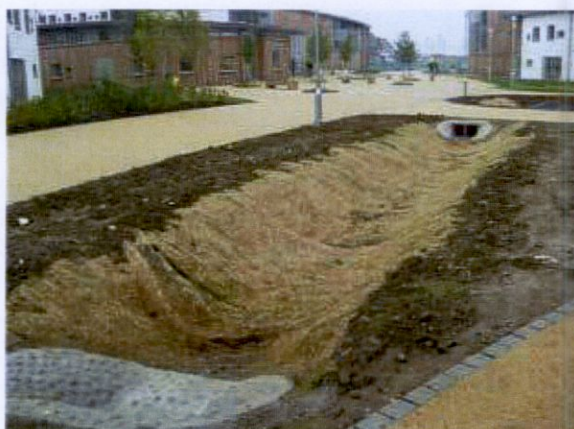
Figure 17.16 Swale during construction showing coir matting used to protect soils from erosion before the establishment of vegetation, University of York (courtesy Arup)
