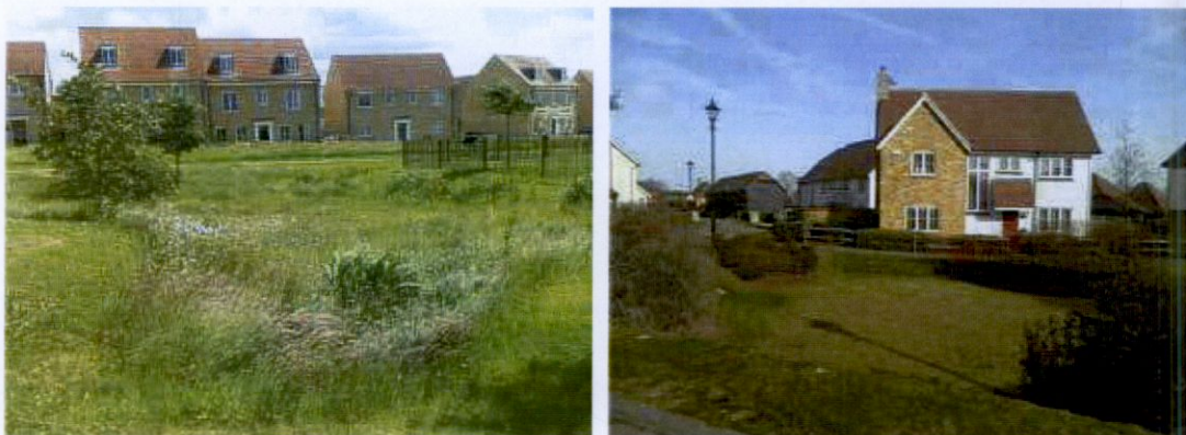
Figure 22.6 Examples of detention basins with easy access for maintenance (courtesy Peterborough City Council and Kent County Council)
