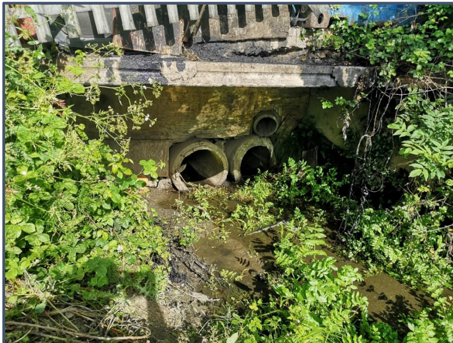
Figure 5-8 Inlet to twin-pipe culvert
