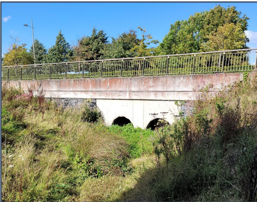
Figure 5-7 Upstream View of Culvert under Park Road
