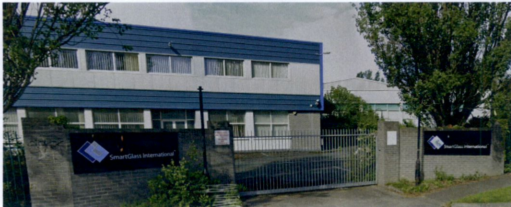
Figure 3 - Existing Site Entrance and Commercial Building Planning for Demolition
