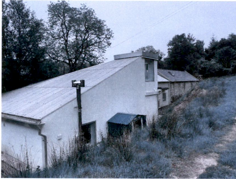
View looking south-east towards the rear of the dwelling
