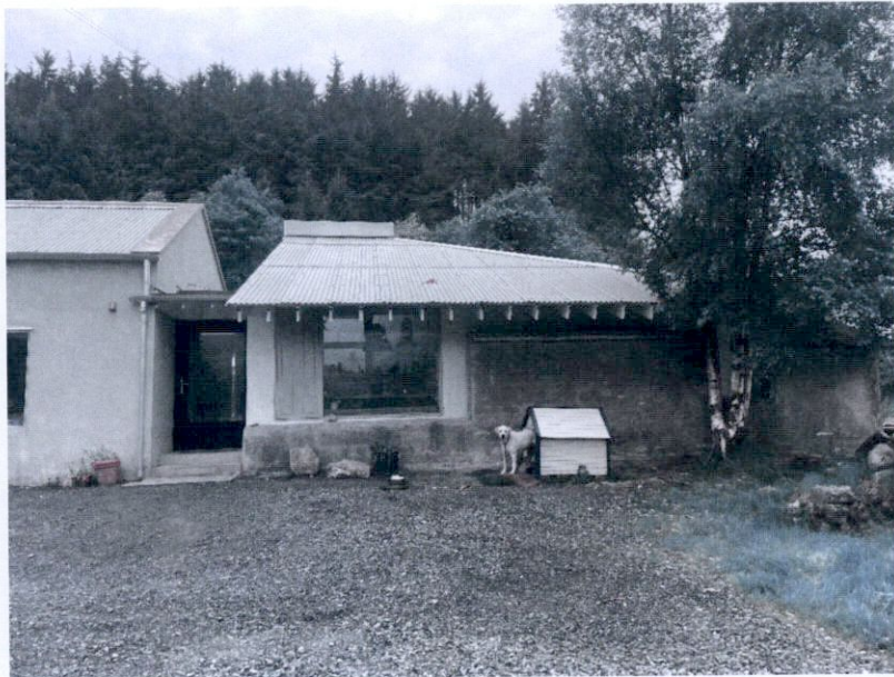
View of the northern part of the renovated cottage
