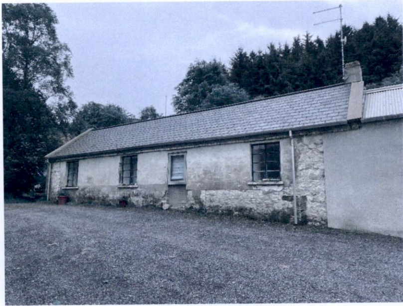
View of the partially renovated cottage with slate and corrugated roof
