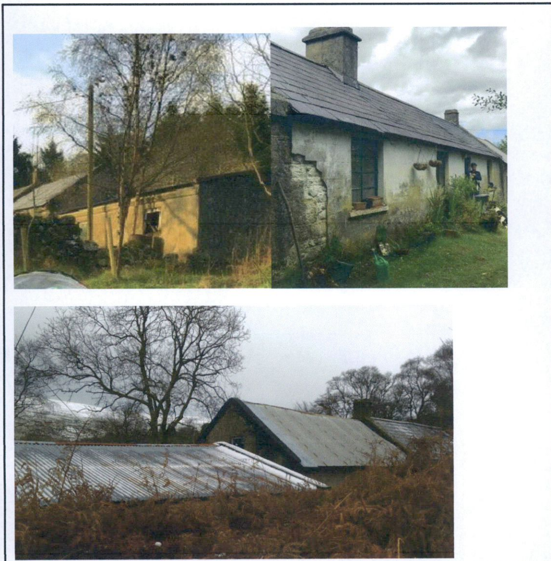
Figure 2.8: Photographs of the Original Structure Prior to any Works
