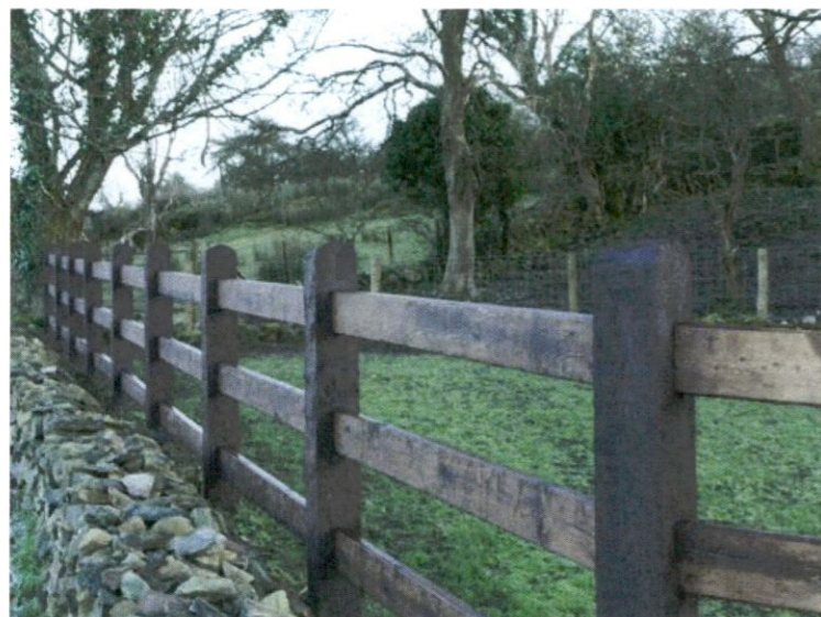
Image showing Timber Fencing
